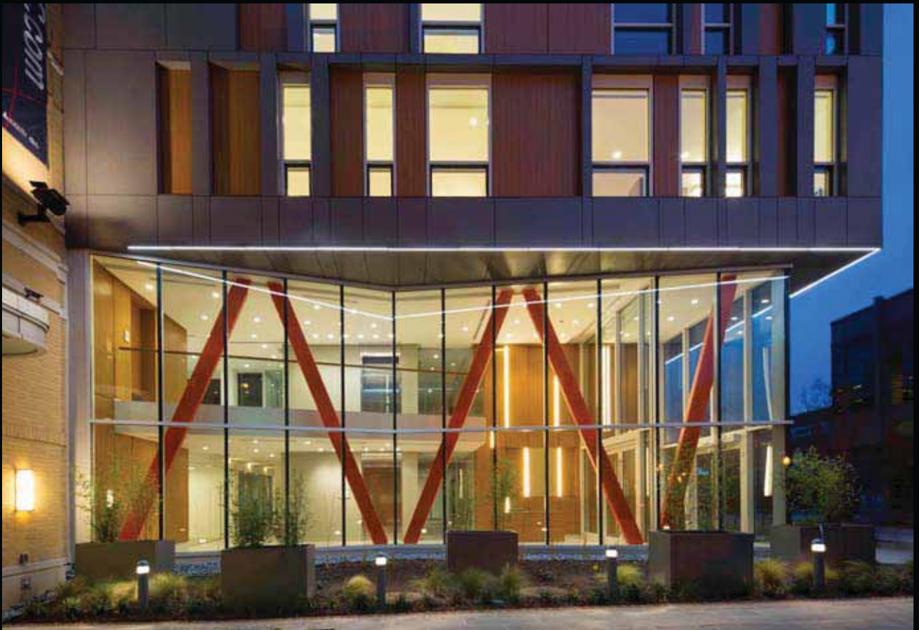
VIEW FROM NEIGHBORING COURTYARD
