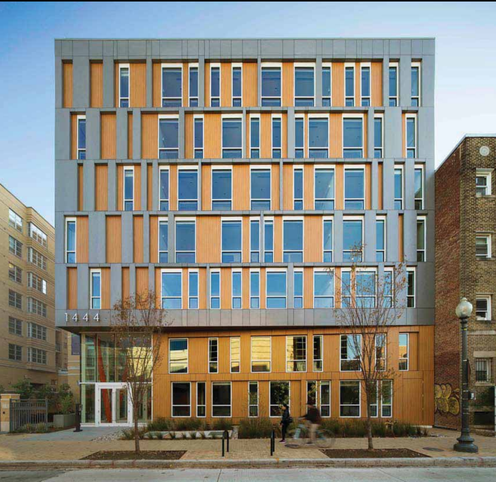
IRVING STREET NW FACADE
