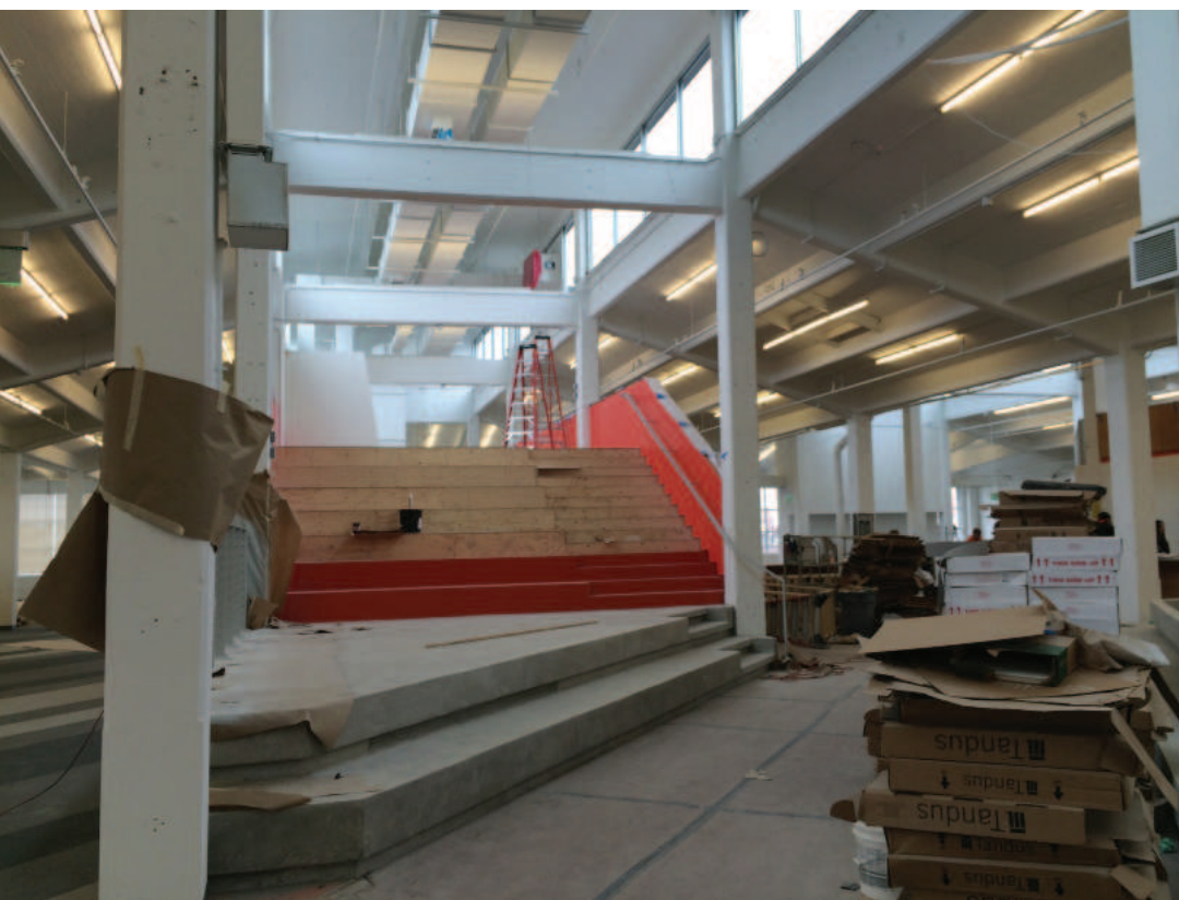
EXPANSIVE EXISTING FLOOR PLATES AND LIGHT MONITORS
