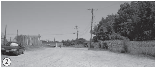
EXISTING: INDUSTRIAL SITE WITH CULVERTED CREEK BELOW
