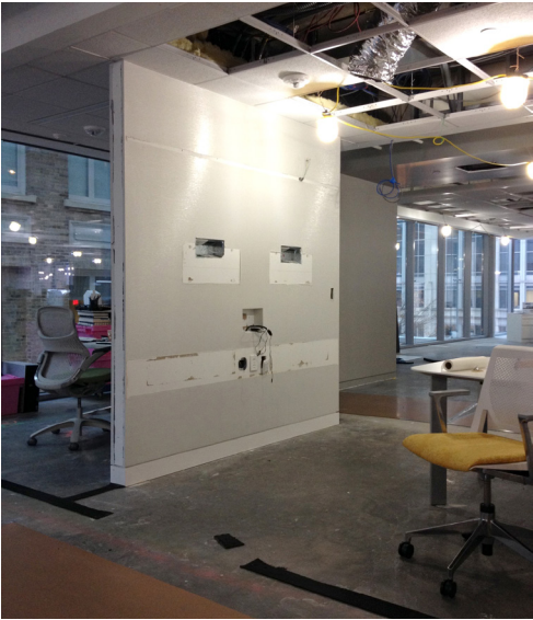
Deconstruction of the Huddle Room
