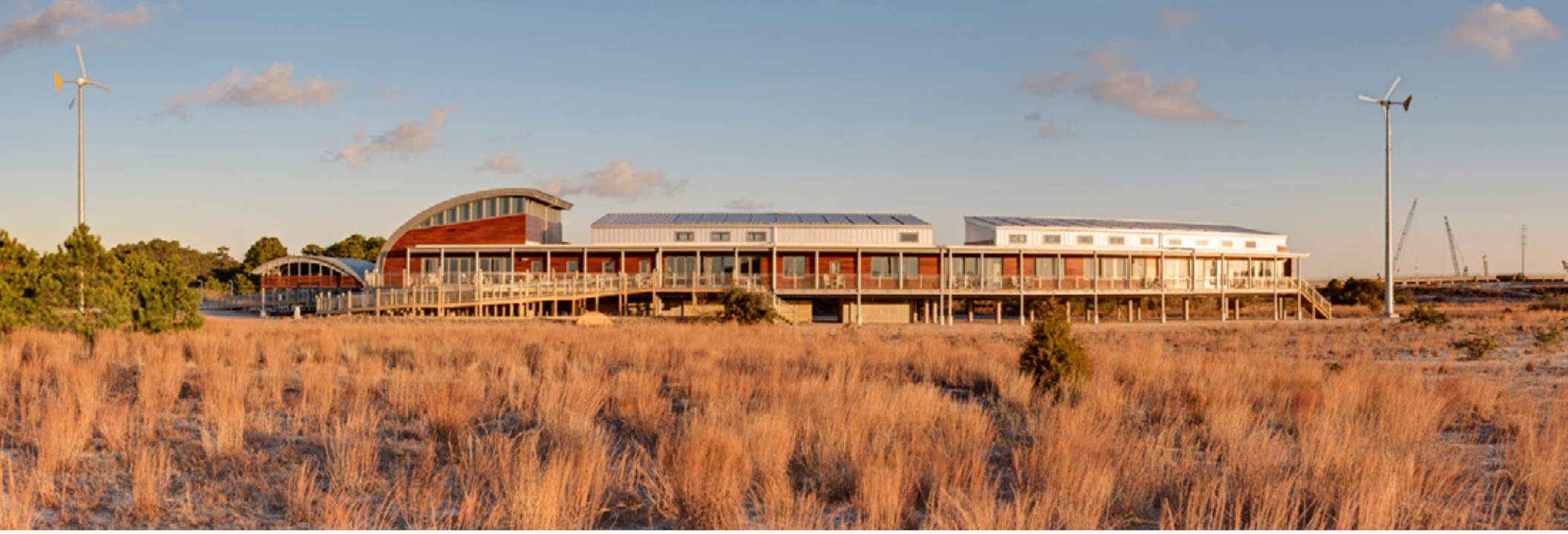
View from the south showing roof-mounted photovoltaics and 2 wind turbines "book-ending" the design.
