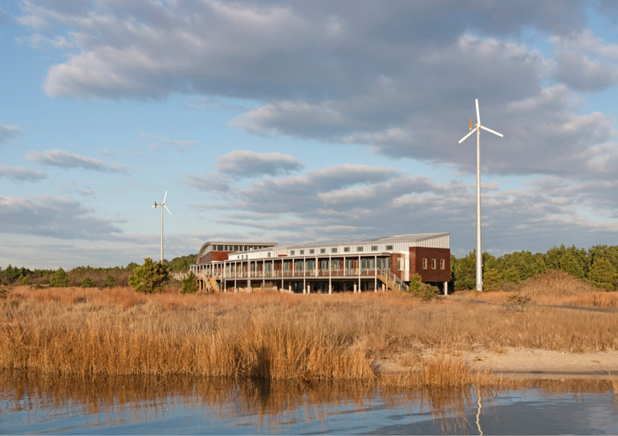
View from the dock looking to the north-west
