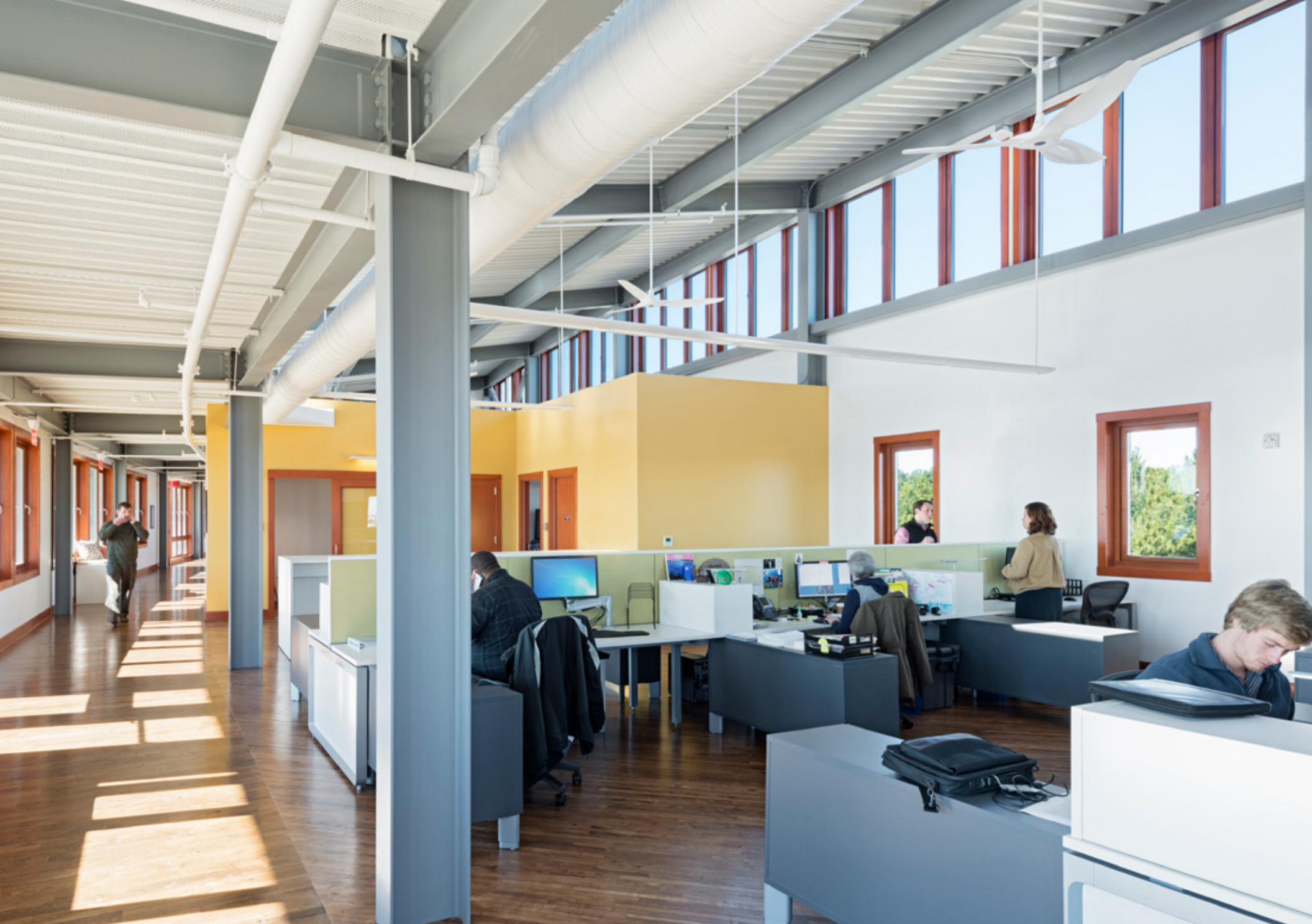
View of open office areas showing northern clerestories that provide ample daylight. The south facing corridor is dappled with light while buffering the office area from glare. Ceiling fans promote airflow during the natural ventilation season.
