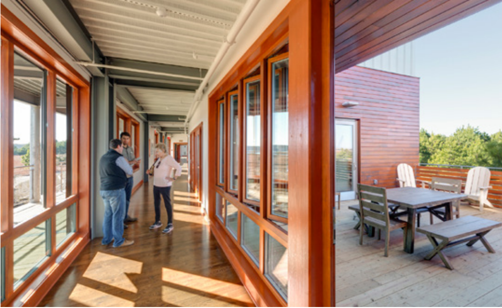
View of the south hallway and the "dog-trot" which enhances natural ventilation.
