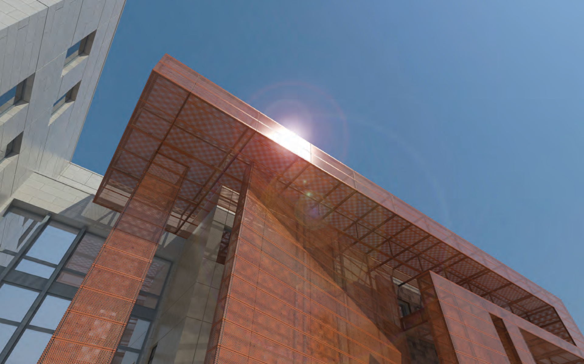
NEW EMBASSY COMPOUND Nouakchott, Mauritania
