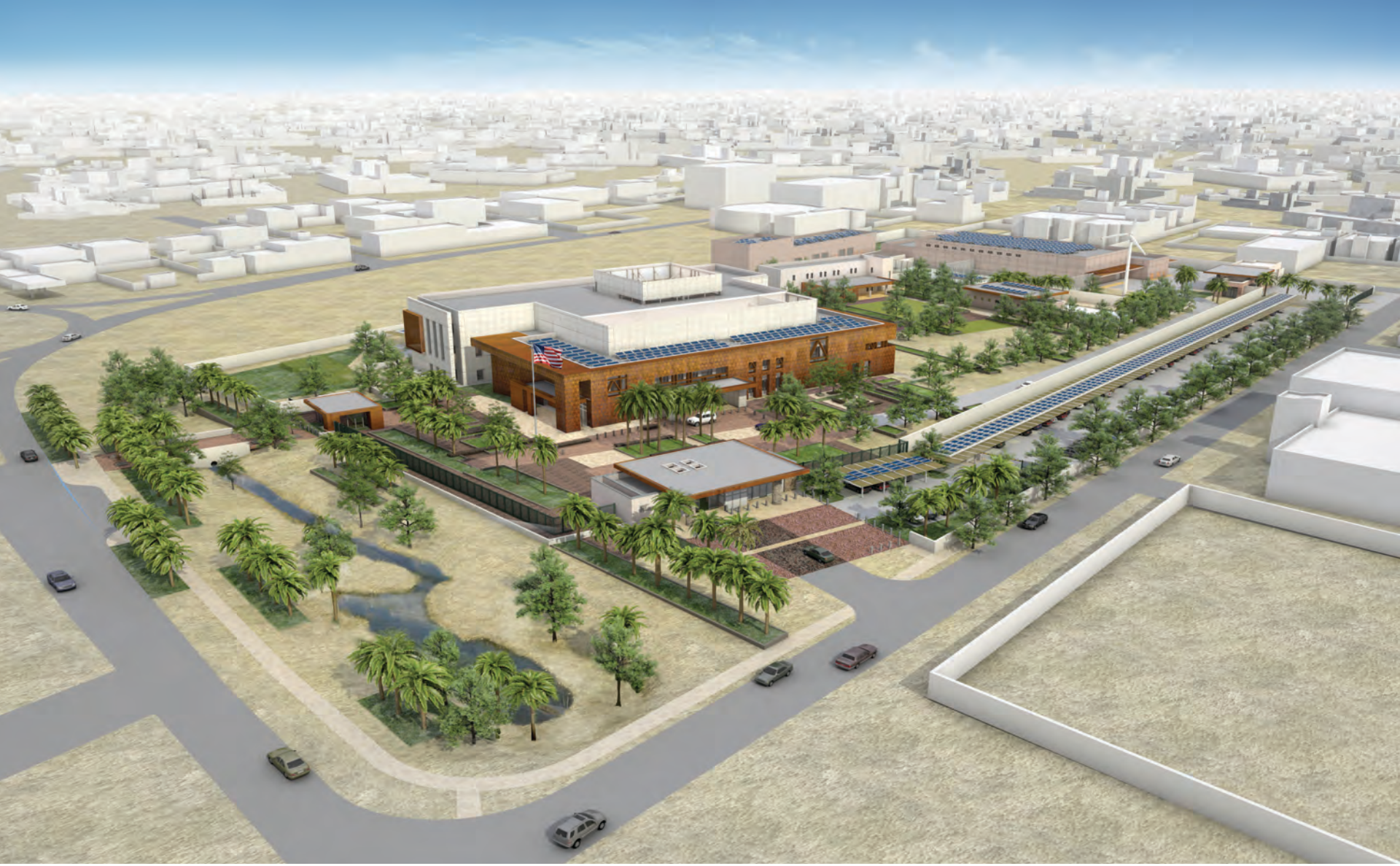
NEW EMBASSY COMPOUND Nouakchott, Mauritania
