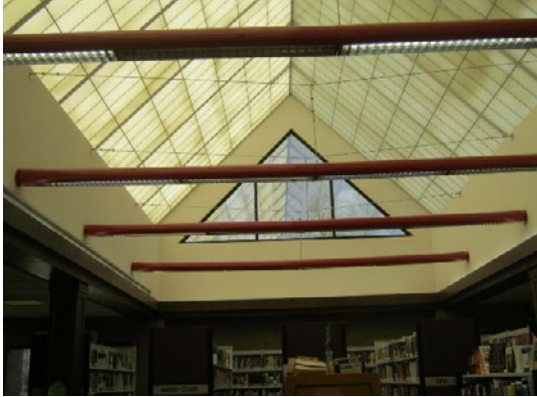
Before — Dark spaces with dim Kalwall skylights.
