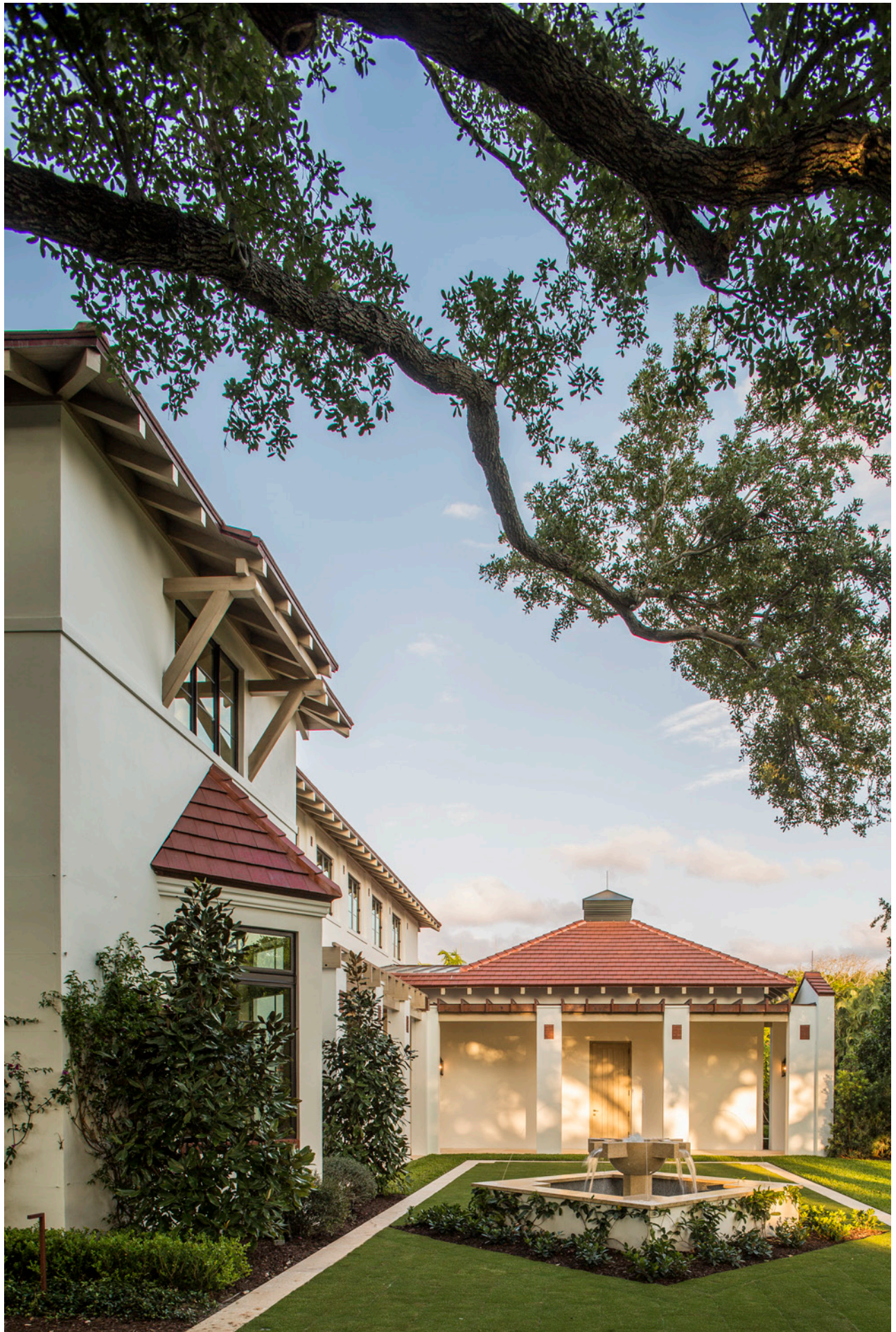
ENTRY GARDEN AND GARAGE/LOGGIA BEYOND
