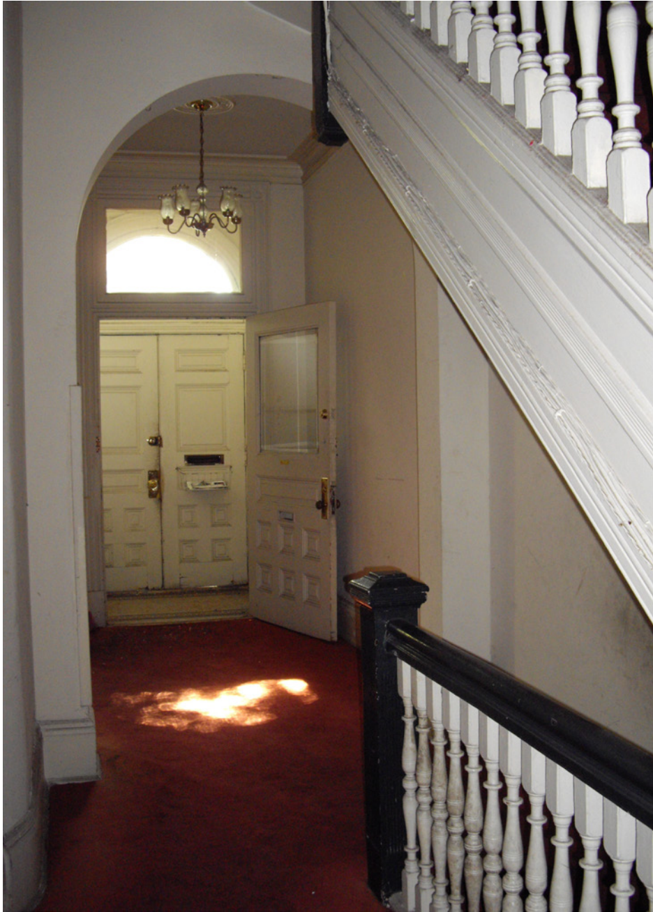
EXISTING STAIR HALL AND ENTRY
