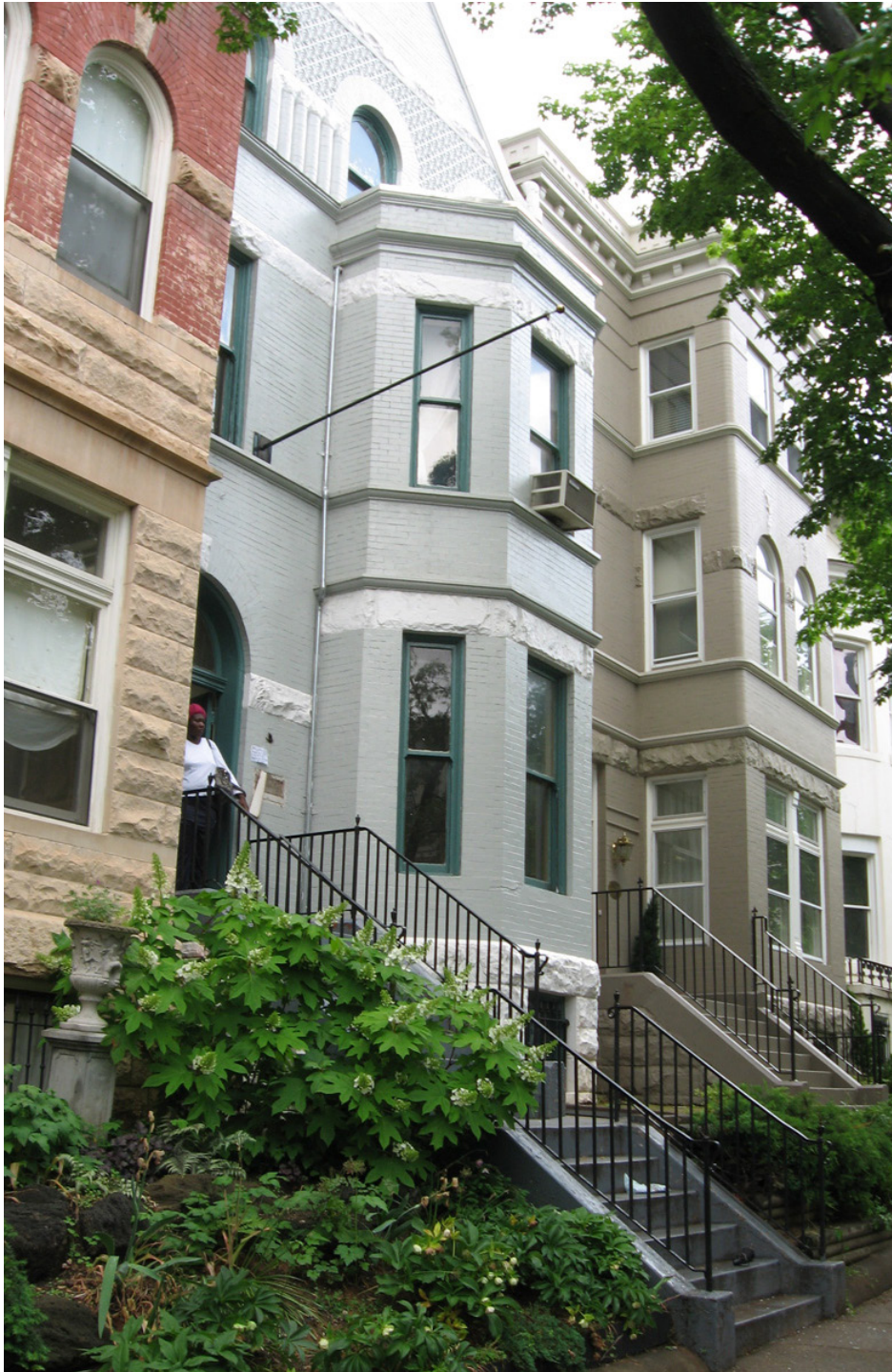
EXISTING FRONT FACADE
