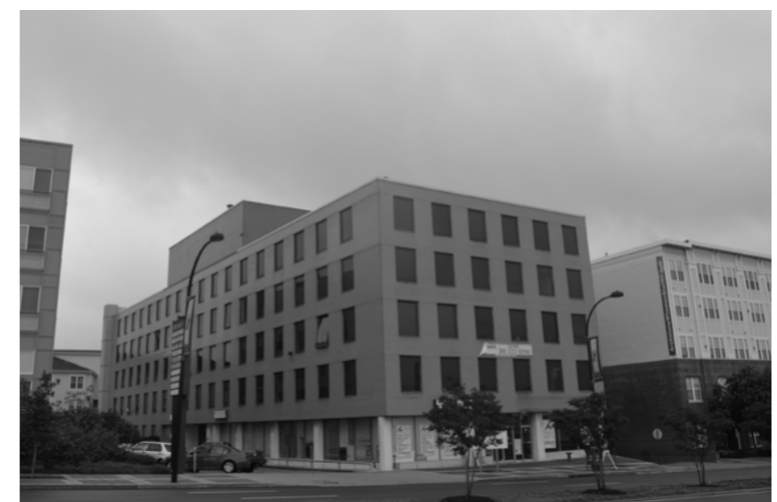
ABOVE The existing 5-Story, 1960s office building
