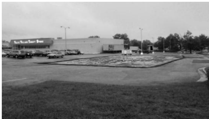
EXISTING VACANT SITE
