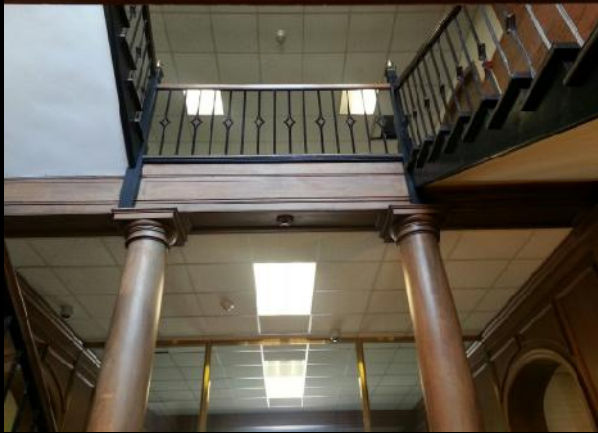
Existing Main Stair
