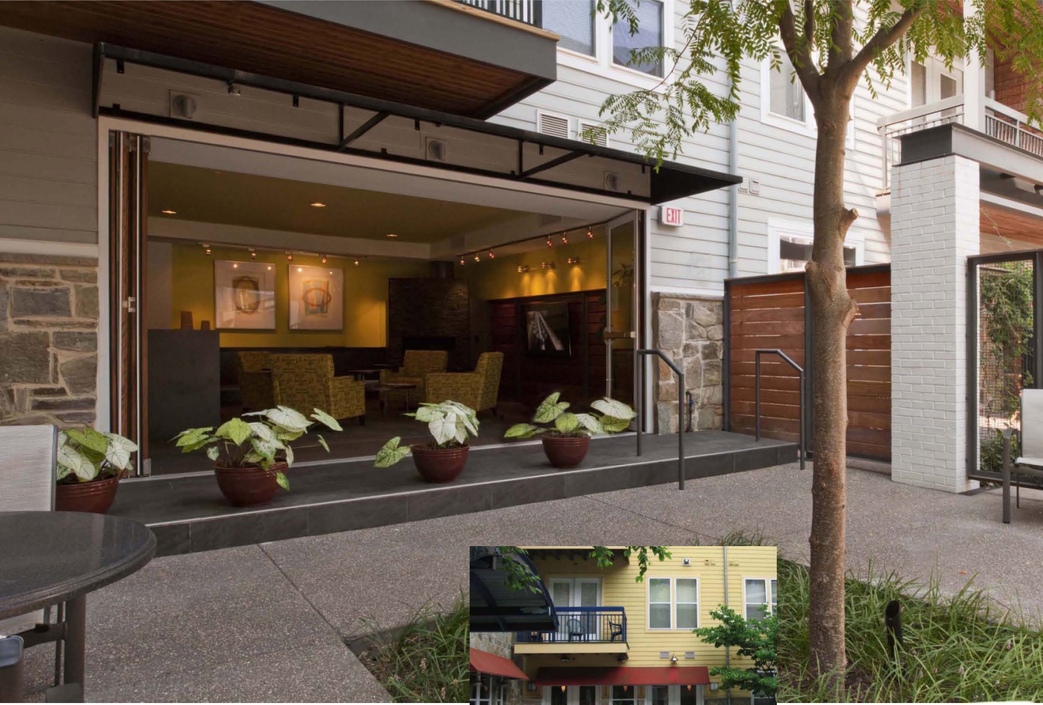
Folding glass walls allow lobby and cafe to fully open to the courtyard.
