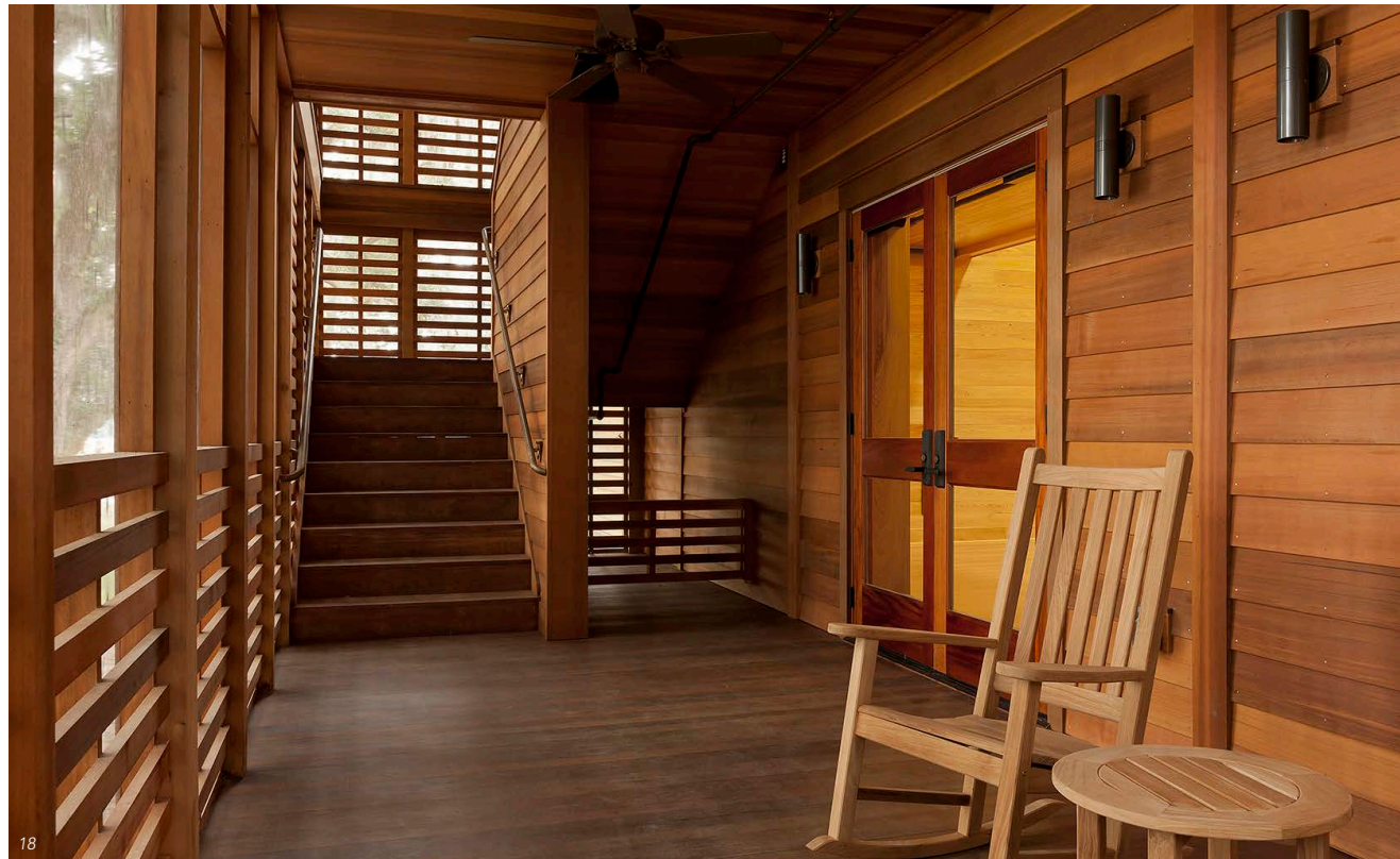
18 View of lower porch; stair connects lower and upper levels
