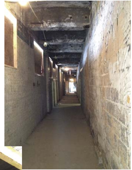
Existing service corridor (1)
