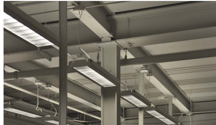
Detail of lighting and power drops (above, top) and interior elevation (below)
