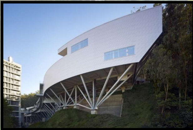
RAY AND DAGMAR DOLBY REGENERATI ON MEDICINE BUILDING IN SAN FRANCISCO, CA
