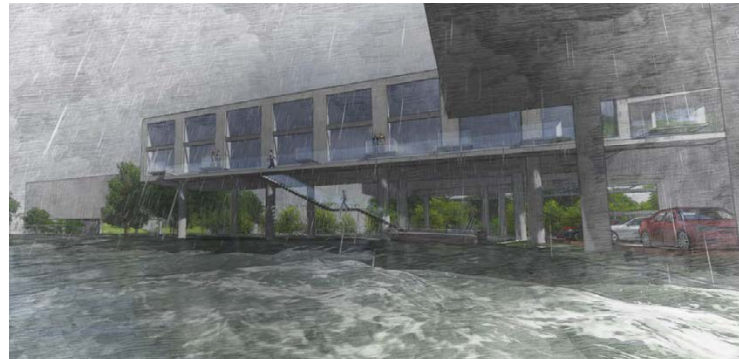
8' Infrastructure Elevated from Significant Storms
