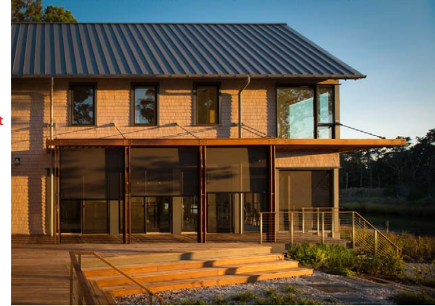
Exterior solar blinds mounted on the outer edge of a pergola create a shaded loggia space and provide protection from the late afternoon sun for the interior rooms.
