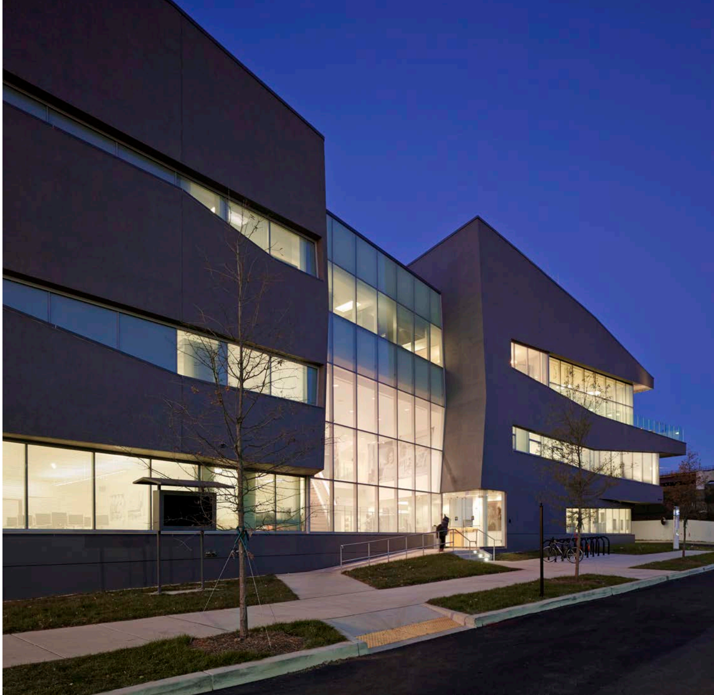
VIEW FROM SOUTH SIDE
