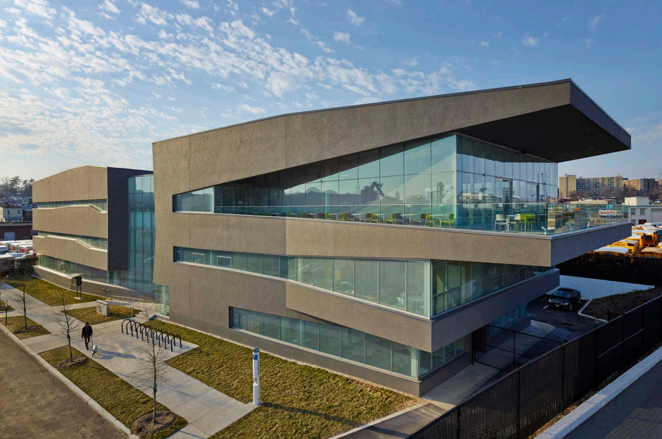
VIEW FROM SOUTH SIDE
