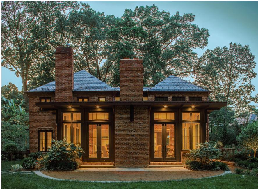
FAMILY ROOM ADDITION
