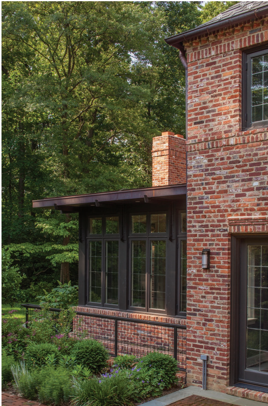
FAMILY ROOM ADDITION
