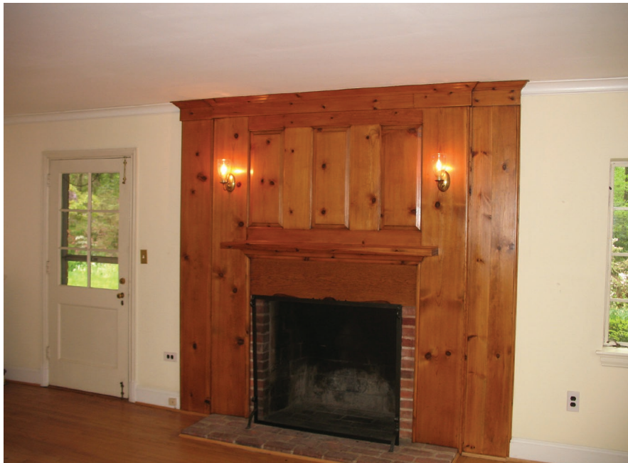
EXISTING LIVING ROOM
