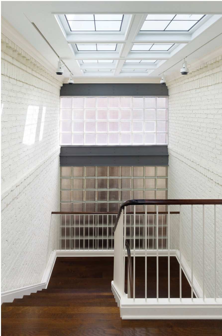
NEW STAIR HALL WITH GLASS BLOCK WALL BEYOND
