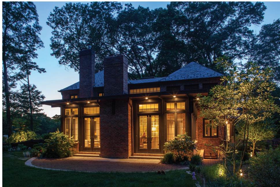
FAMILY ROOM ADDITION
