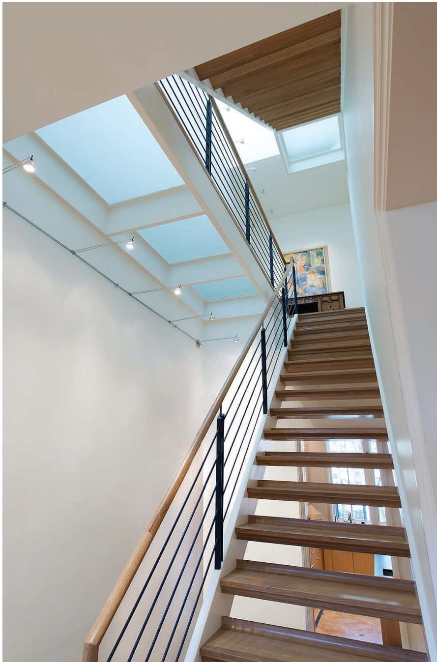
HANDRAIL, TREAD, AND OPEN RISER DETAILS
