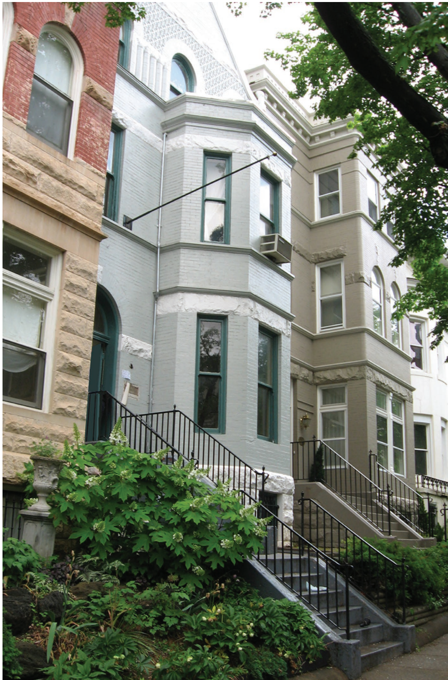
EXISTING FRONT FACADE
