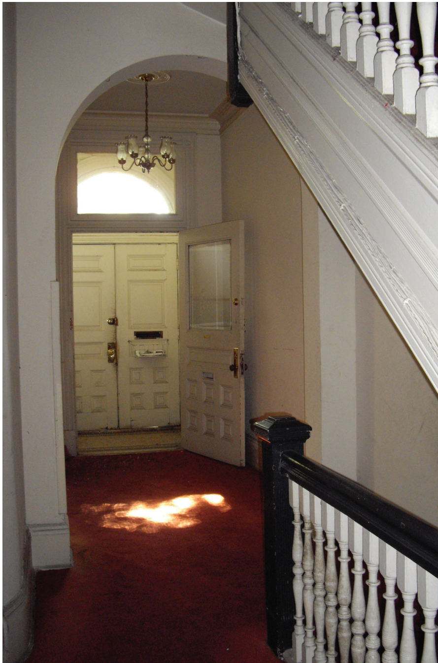
EXISTING STAIR HALL AND ENTRY
