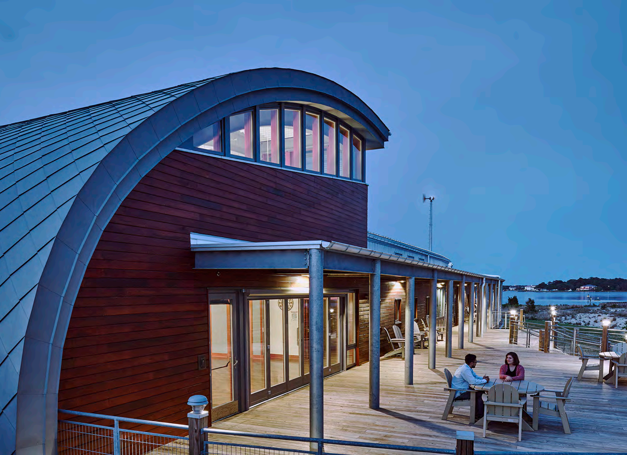
The exterior palette of zinc shingles, sinker-cypress, and galvanized steel reflect the color and forms of the site.
