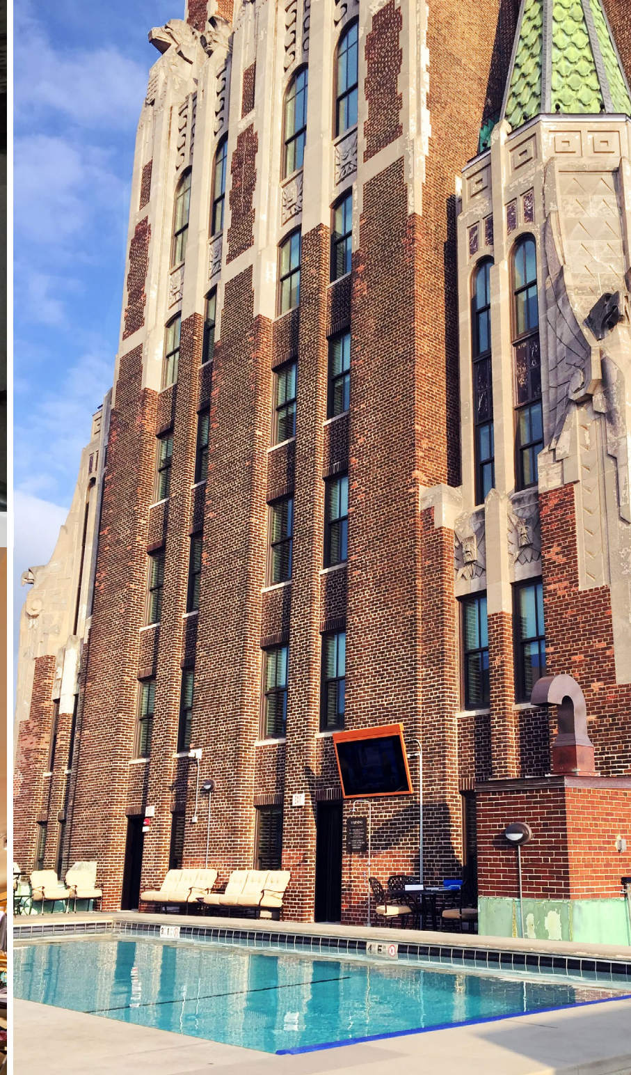
22nd Floor Rooftop Pool An obsolete water tank was converted into an swimming pool.
