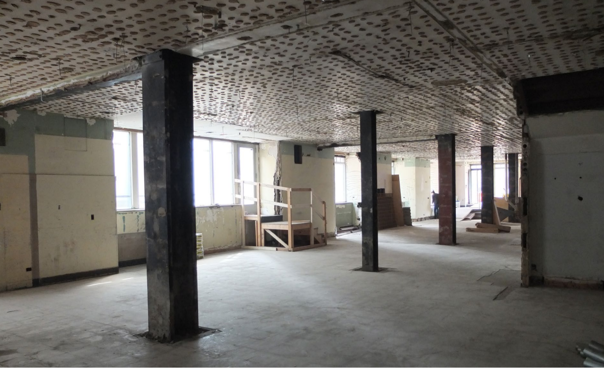
Under Armour Retail Store (before)
