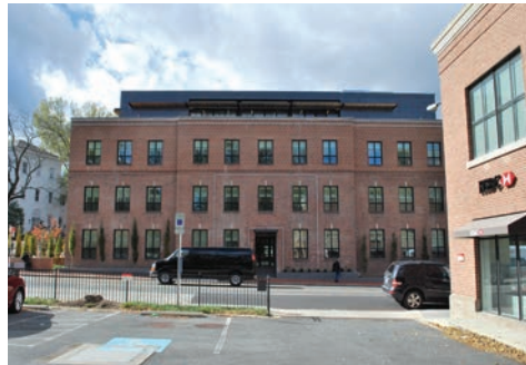
VIEW ON WISCONSIN AVE., COMMERCIAL DISTRICT
