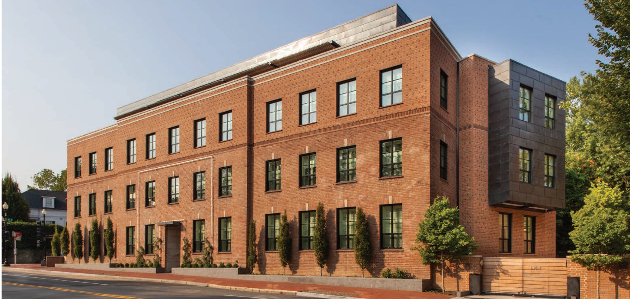
RENOVATED FELLOWSHIP HOUSE - AFTER
