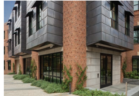
VIEW FROM INTERIOR COURTYARD OF RESIDENTIAL BAYS
