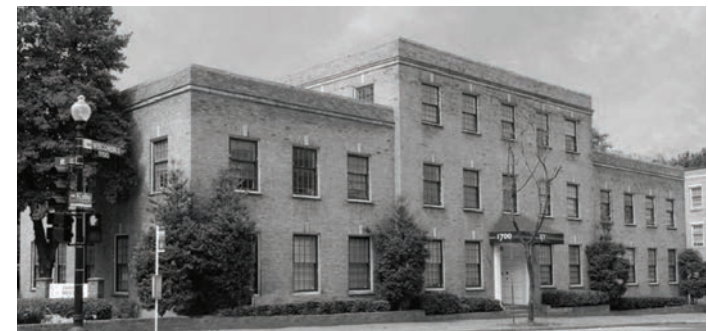
ORIGINAL BUILDING PRIOR TO RENOVATION - BEFORE
