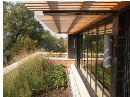
INTENSIVE GREEN ROOF
