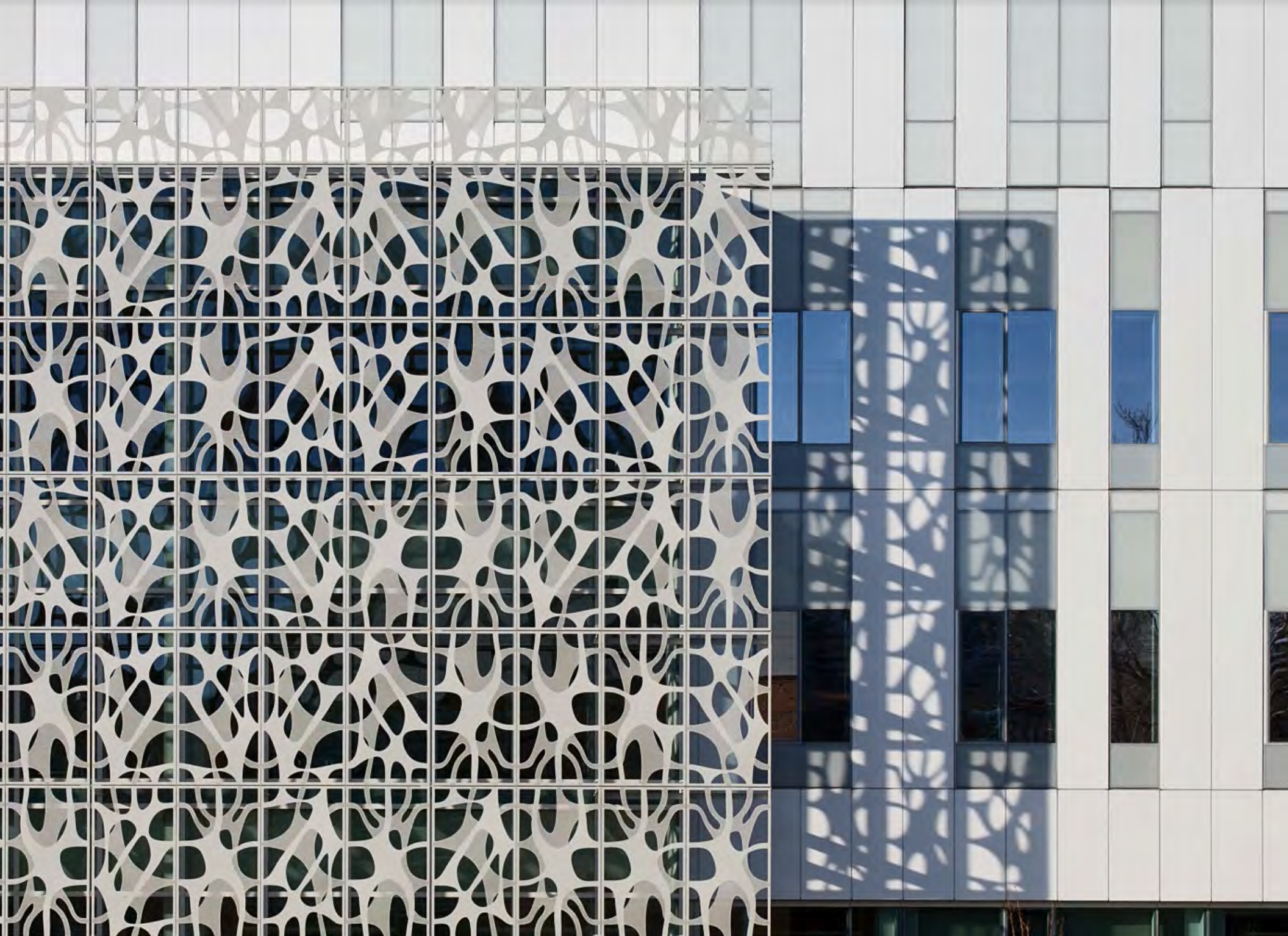
The iconic south facing scrim heps define the life sciences precinct. The sunscreen creates ever changing shadows on the interior and exterior of the building.
