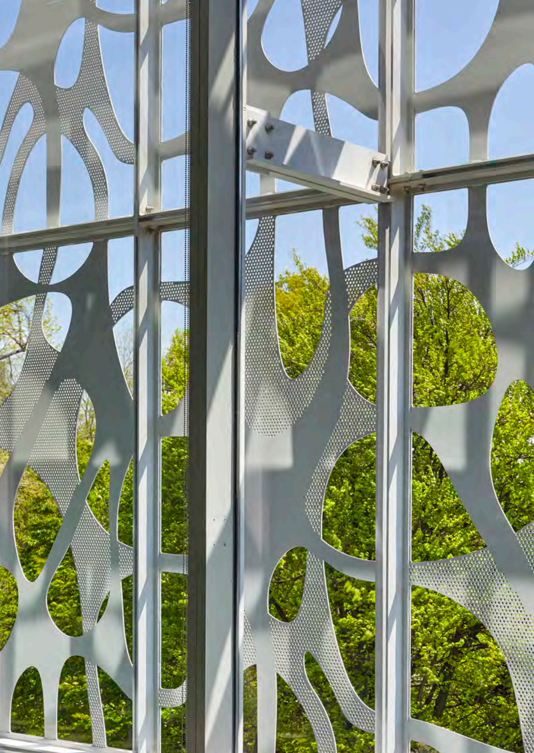
As a reference to biology using the absolute minimum to create complexity, and to maximize the efficiency of construction, the sunscreen panels were configured with only two patterns which could be installed in four configurations totaling eight variations. The panels were designed to connect at the same points, no matter how the panels were configured. The sunscreen reduces heat loads and glare on the south facing glass but still allows for expansive views.
