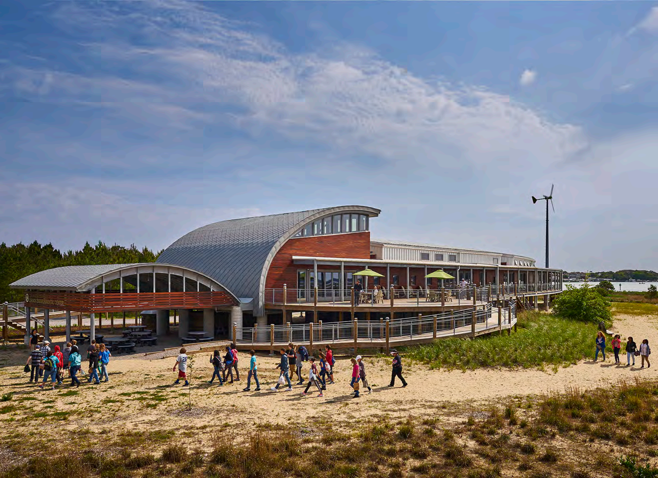
View of the Center from the southwest, during a field trip. The Center's low profile and curving forms integrate with its sensitive site.
