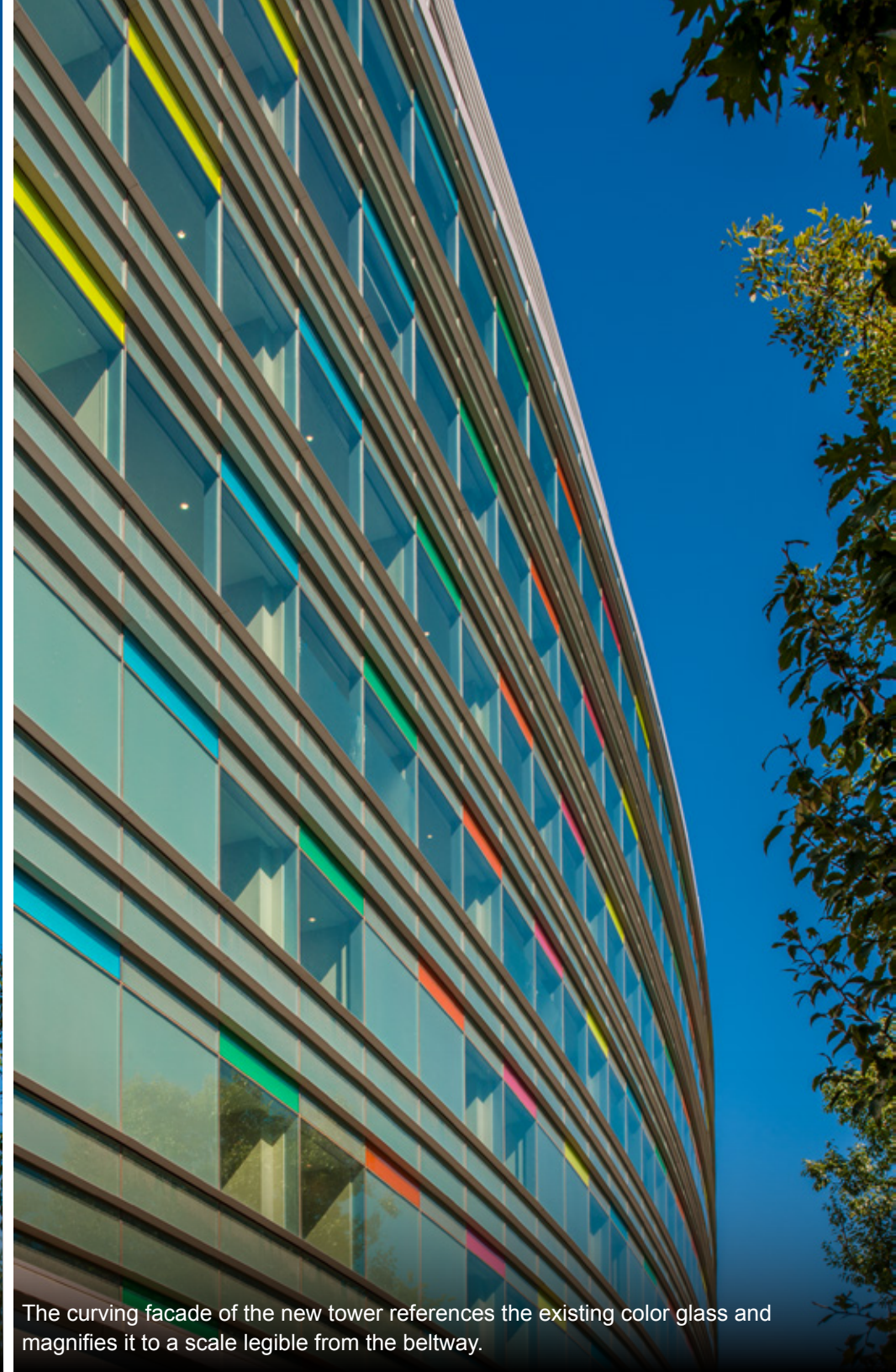
The curtain wall was acoustically designed to ensure patient comfort and mitigate noise generated by beltway traffic.
