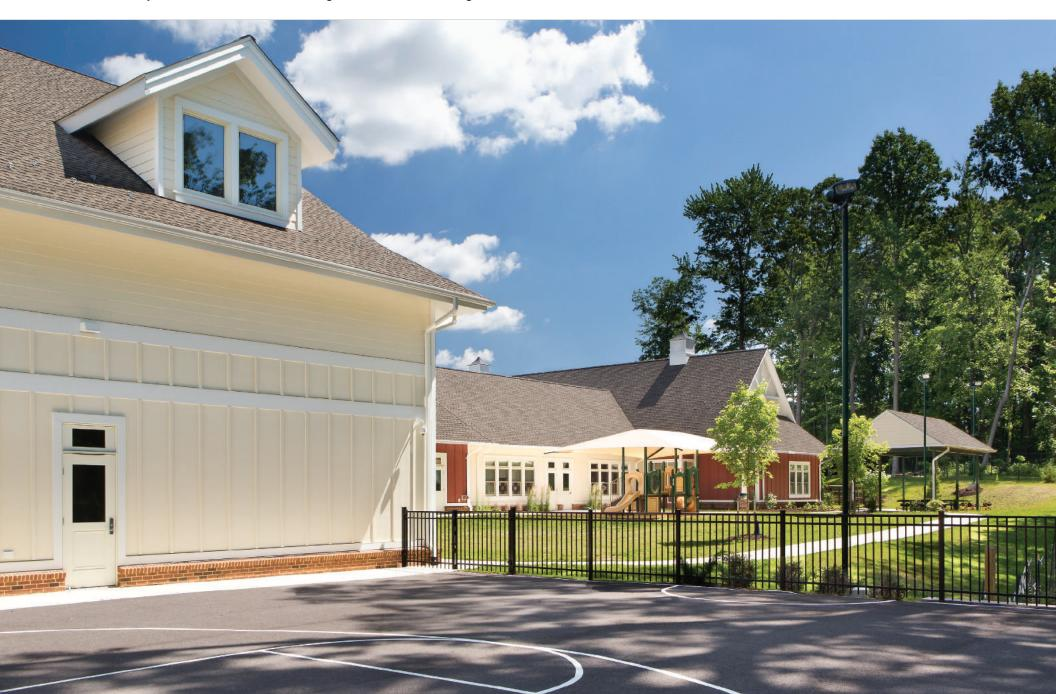
For the annex building, the steep sloped roof rotates differently from the main daycare building and a high clerestory dormer window is included, providing visual clues that a unique curriculum is housed within. The increased roof height also provides space for an elementary-sized indoor basketball court in the rear half of the building.
