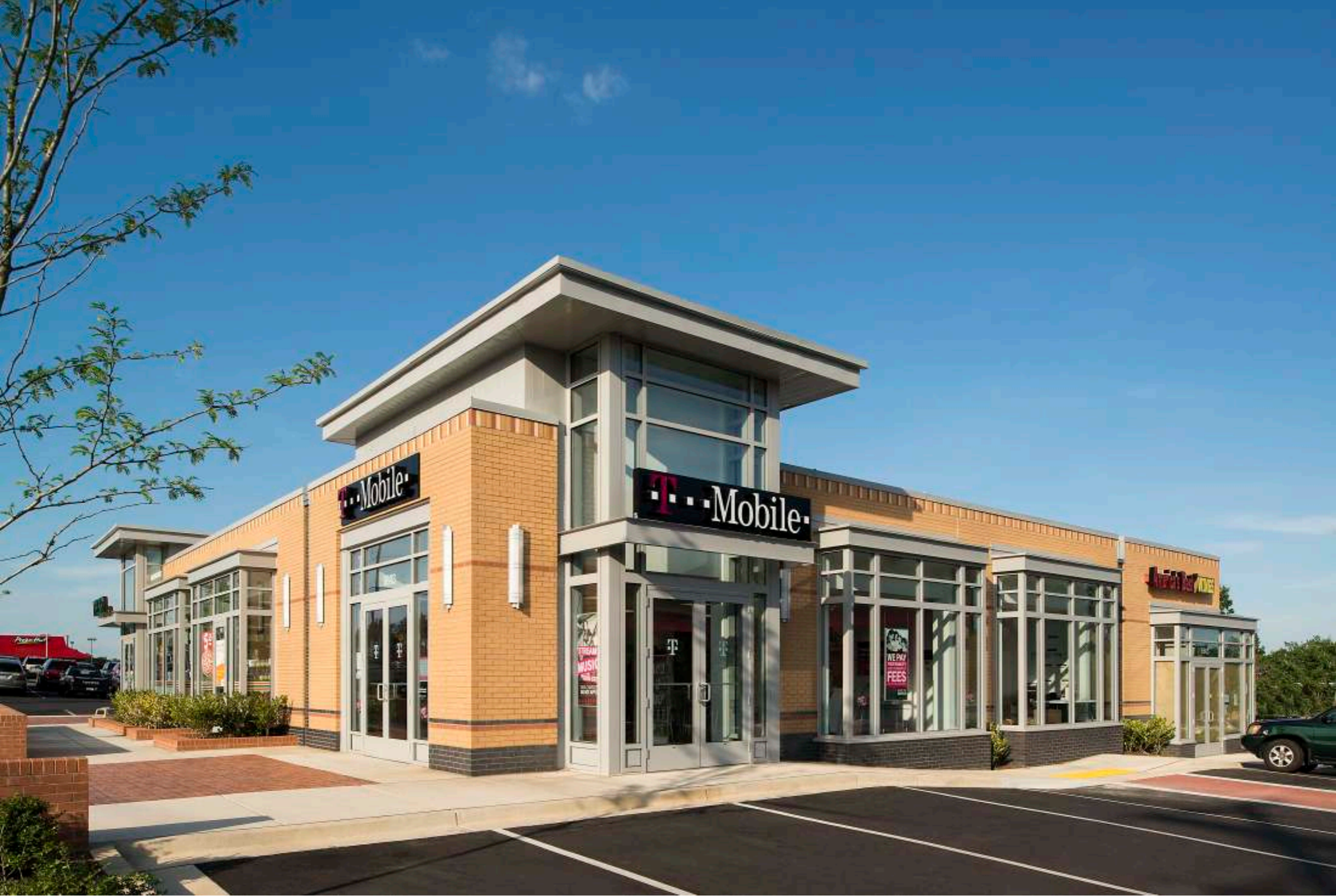
Cooper Lane Road facade, facing east
