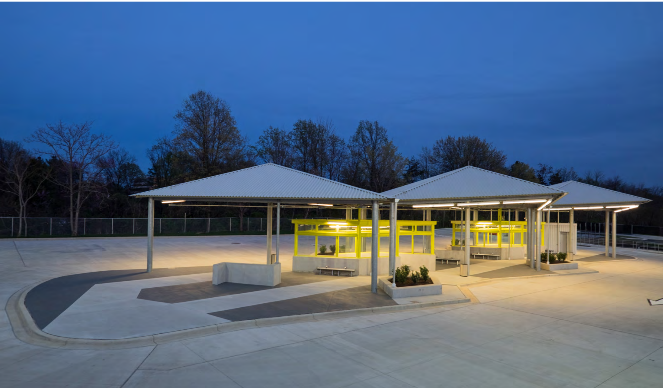
View Looking South East from Bus Exit Ramp
