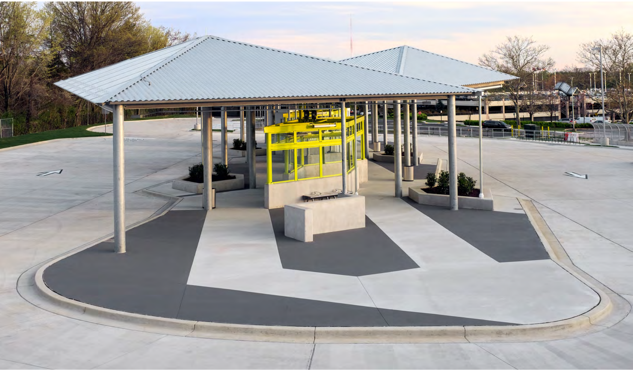
View Looking South from Westlake Terrace Overpass
