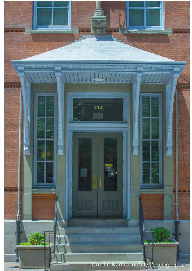
ENTRANCE WORK AFTER
