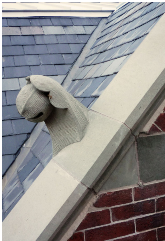
MASONRY WORK AFTER
