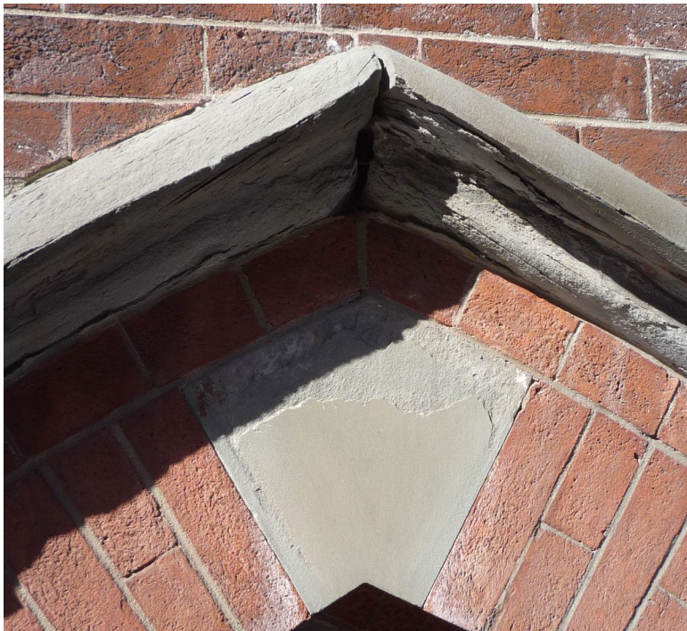
MASONRY WORK BEFORE
