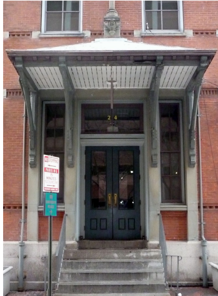
ENTRANCE WORK BEFORE
