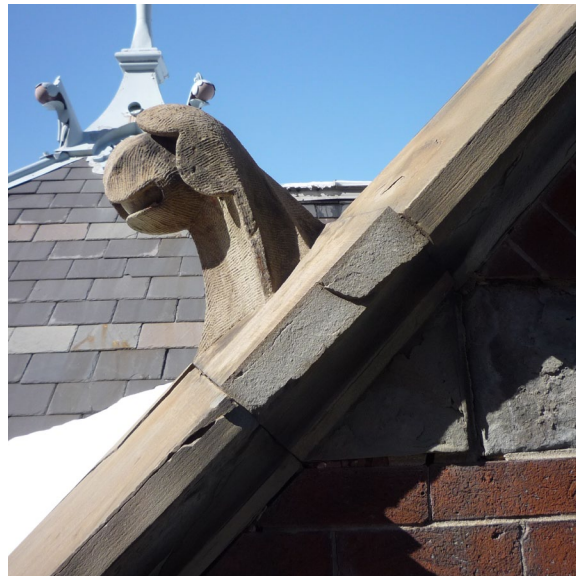
MASONRY WORK BEFORE
