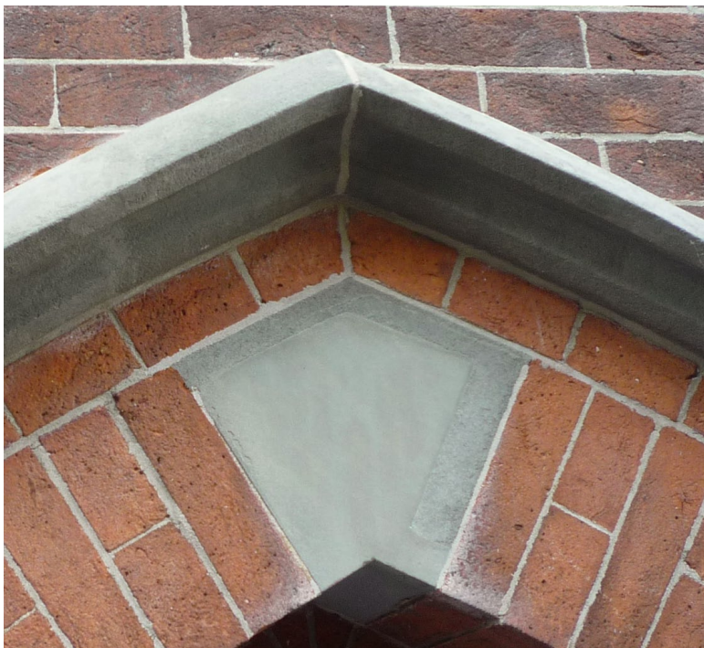
MASONRY WORK AFTER
