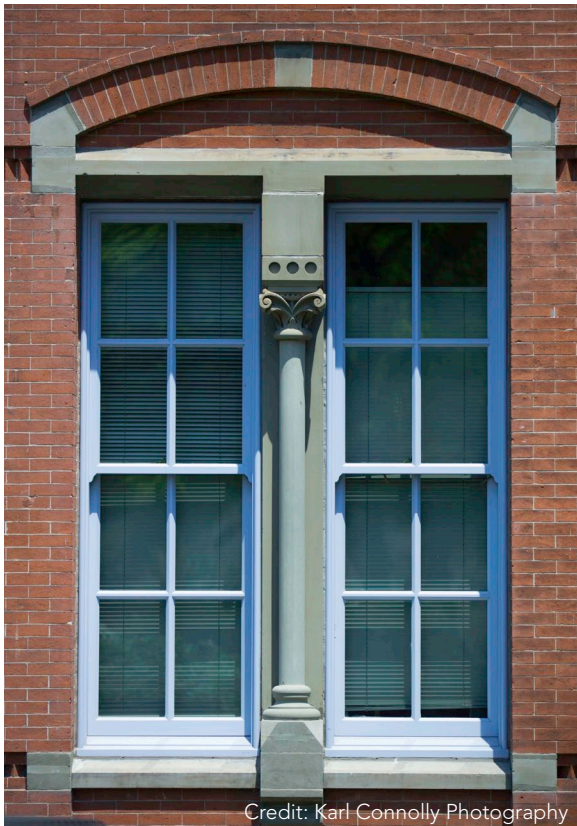
WINDOW/MASONRY WORK AFTER
