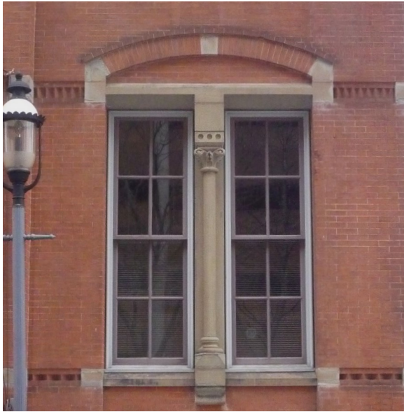
WINDOW/MASONRY WORK BEFORE
