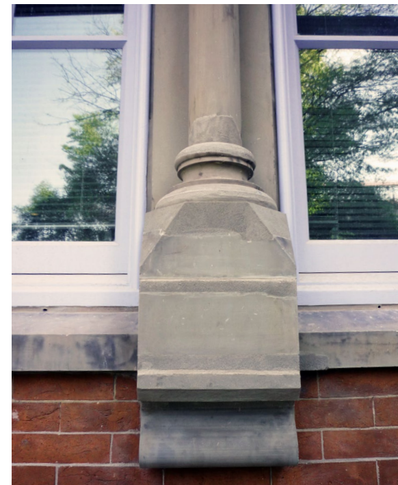
MASONRY/WINDOW WORK AFTER
