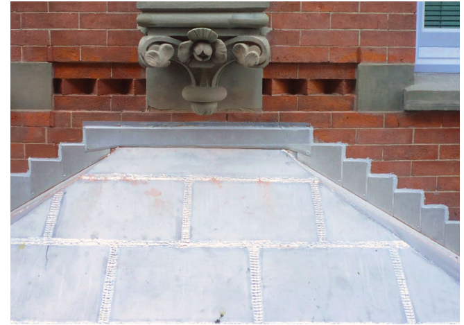
ROOFING/MASONRY WORK AFTER
