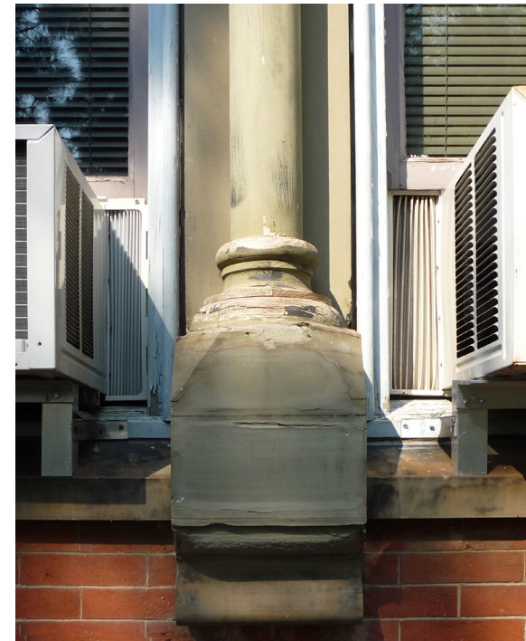
MASONRY/WINDOW WORK BEFORE
