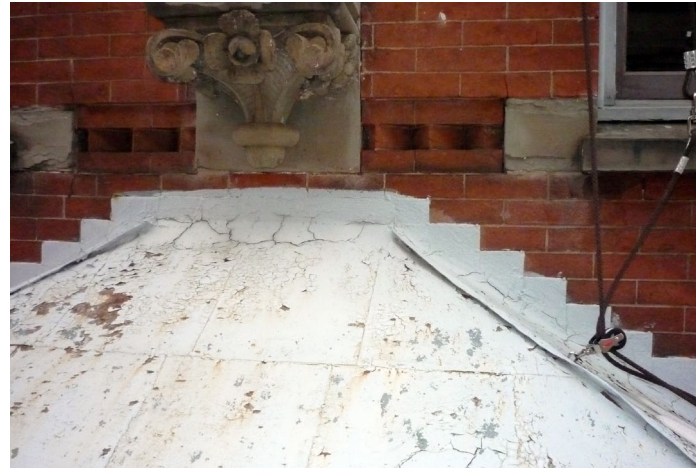
ROOFING/MASONRY WORK BEFORE
