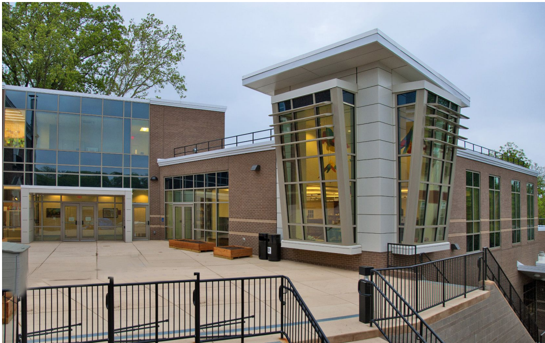
View of completed Media Center and South entrance plaza
