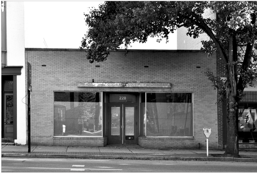
Front of Building (existing conditions)
