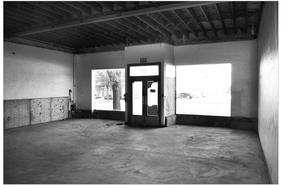
Building Interior (existing conditions)
