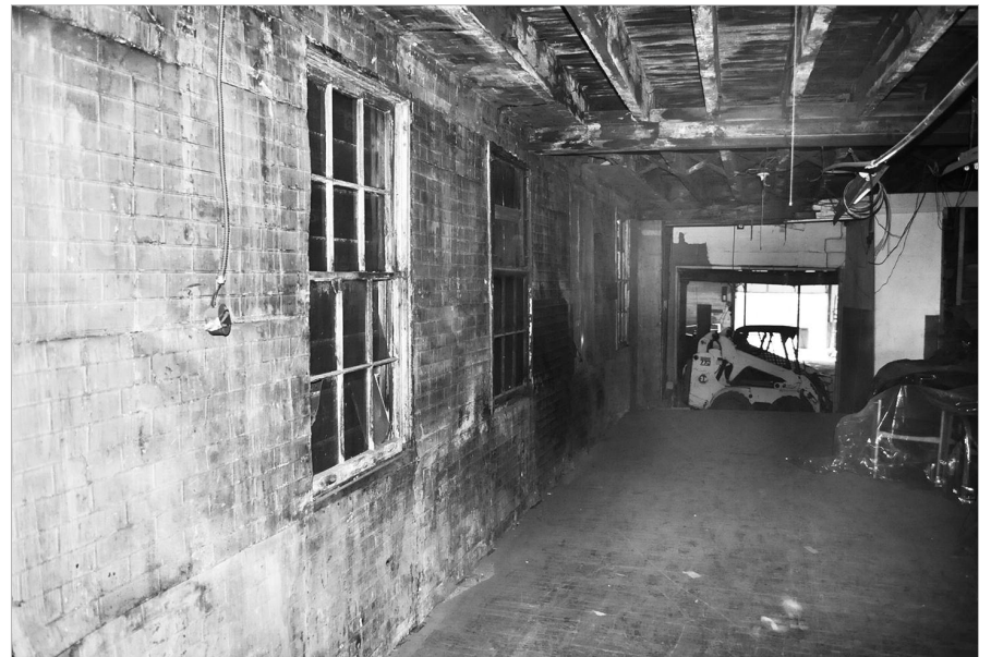
Building Interior (existing conditions)
