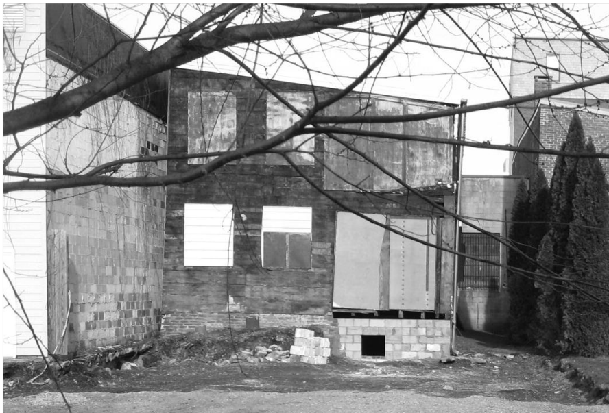
Rear of Building (existing conditions)
