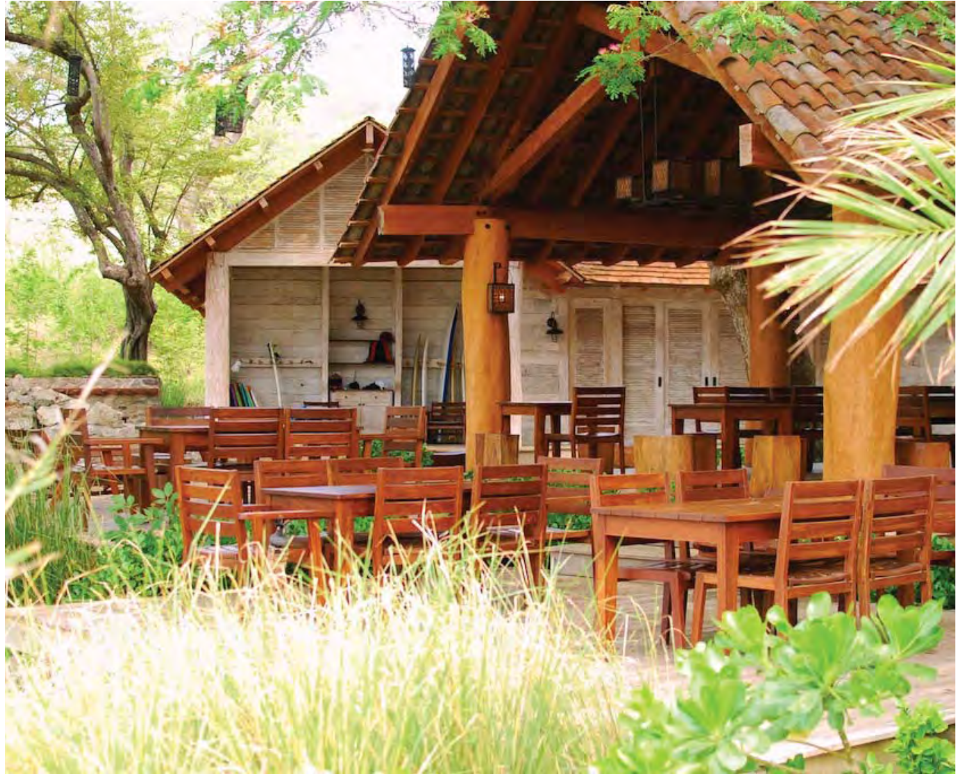
The surf shop and school can be seen as a layer though the open bar pavilion. Large barn doors screen the retail function, while a generous porch provides space for board repair or simply watching the waves.
