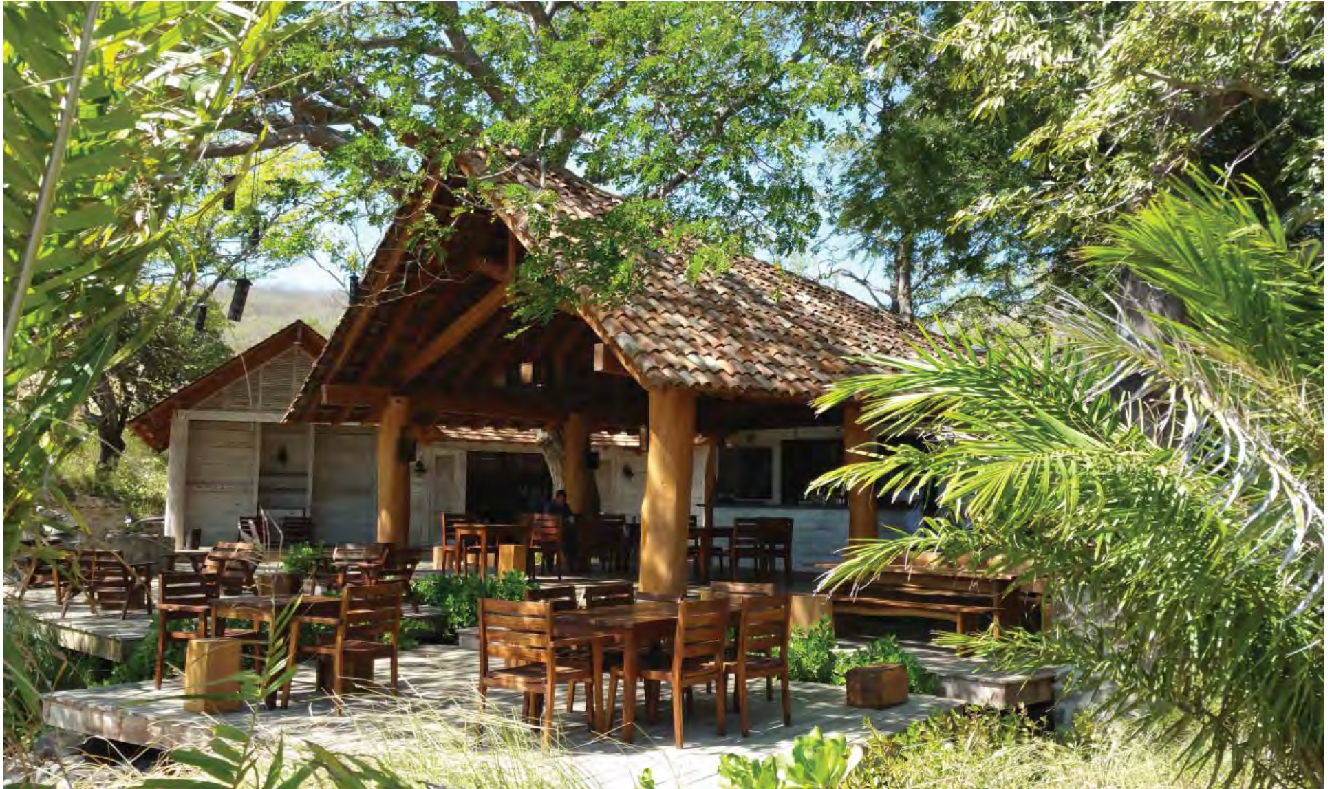
The open bar pavilion filters the view of the surf shop beyond, as both structures nestle into the adjacent vegetation.
