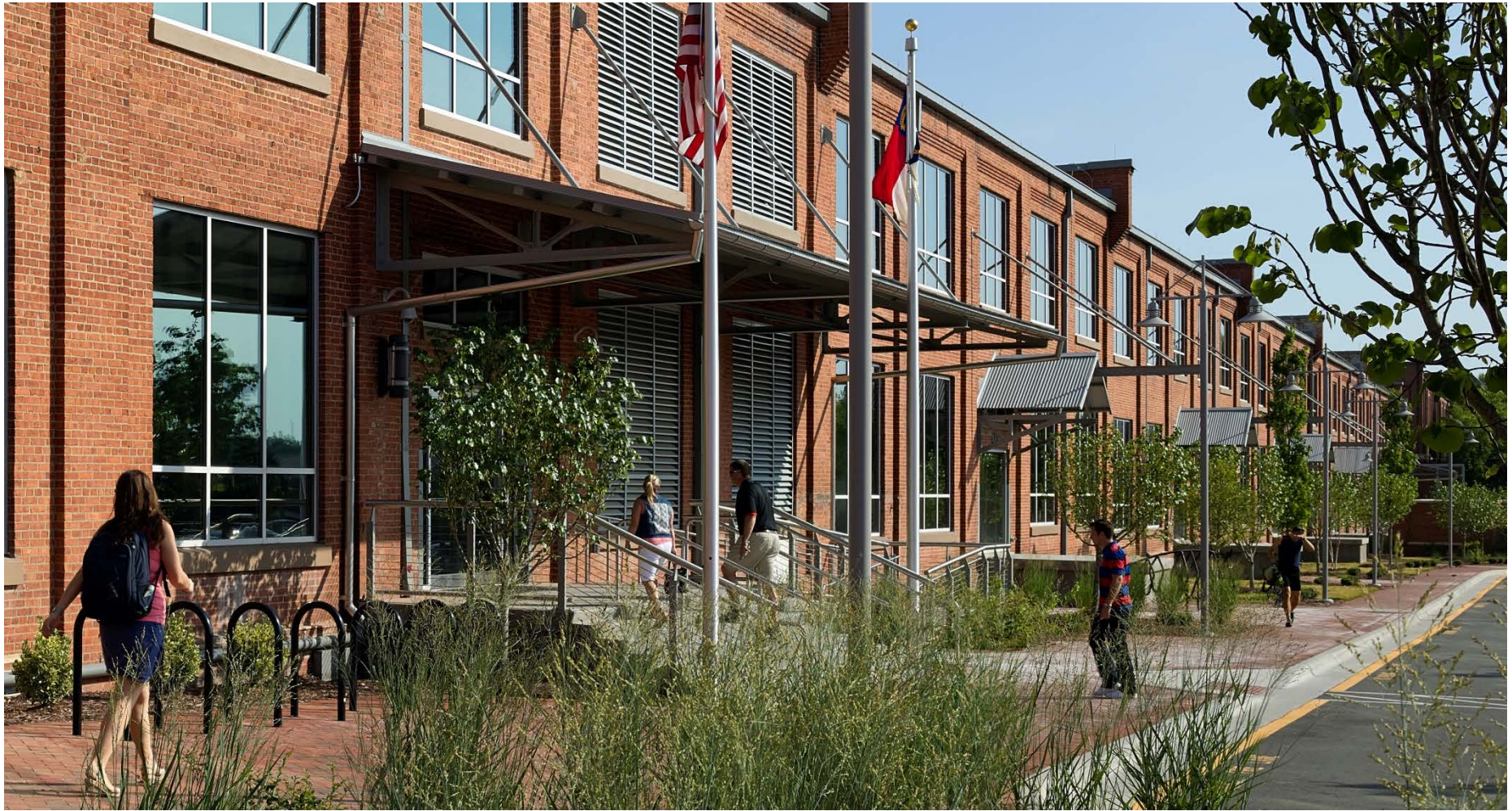
New entrance canopy and stairs with the signature Carmichael louvers, loading platforms and rigging, all restored to invoke the former warehouse district for one of the world's three major tobacco companies.
