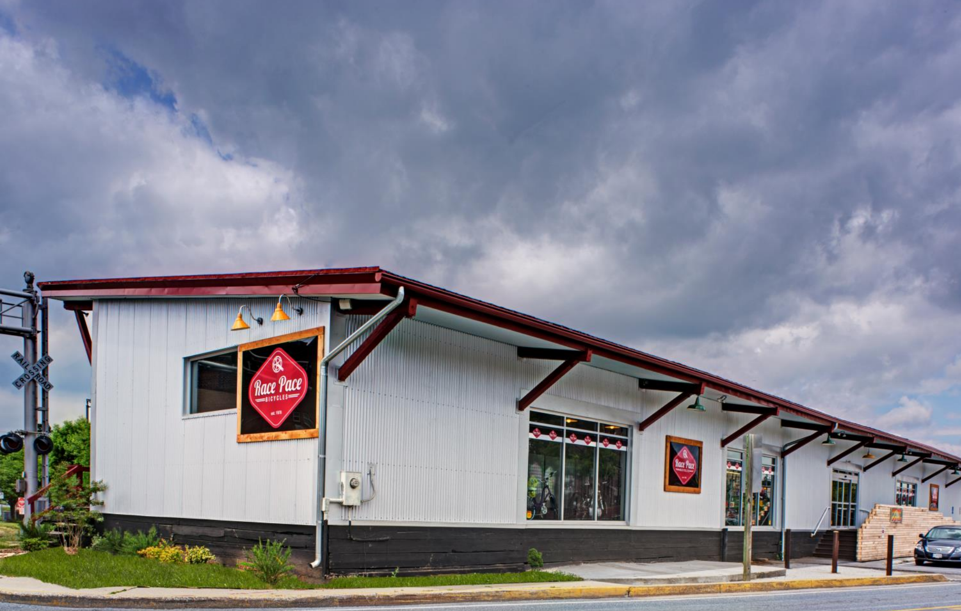
Installed Stanley Automatic Sliding doors at main entrance and service entrance to make it easier for customers to move bikes in and out of the store
