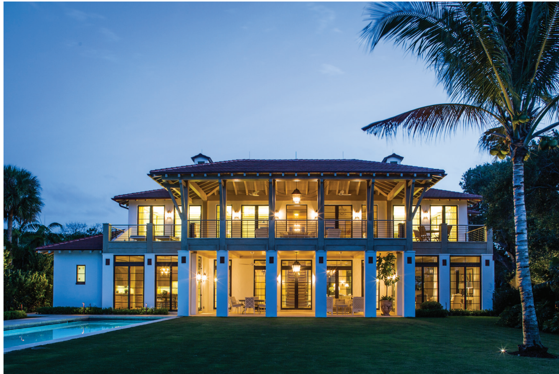
POOLSIDE TERRACE AND NORTH FACADE
