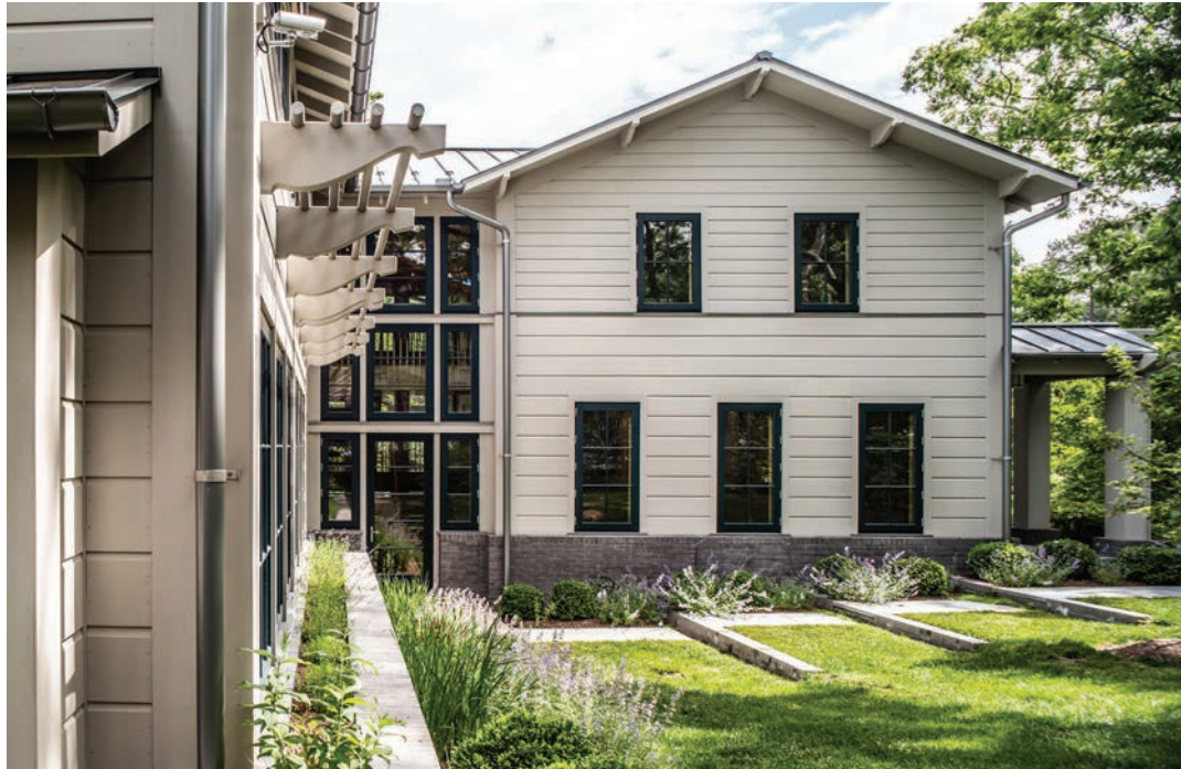
SOUTH FACADE OF FRONT WING WITH STAIR HALL HYPHEN
