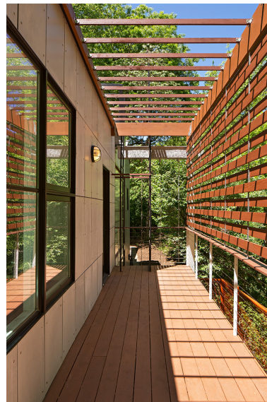
Second floor deck with trellis, large metal gutter and ship ladder to roof.
