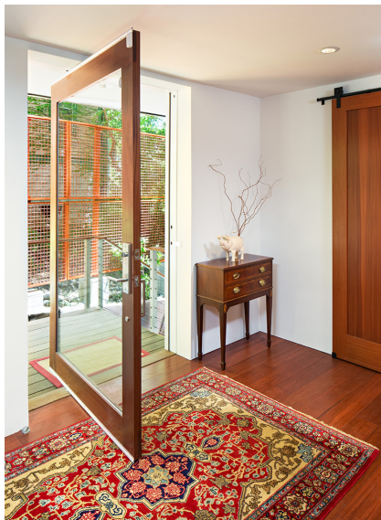
Main entrance pivot glass door.
