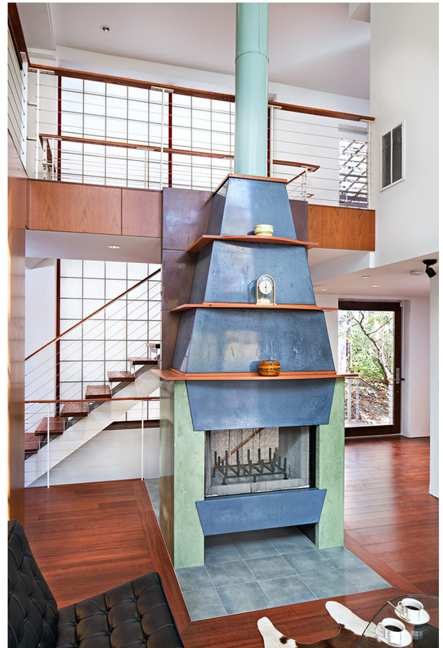
Concrete fireplace with two sides placed on porcelain base in front of the vestibule area with a pivot glass door.
