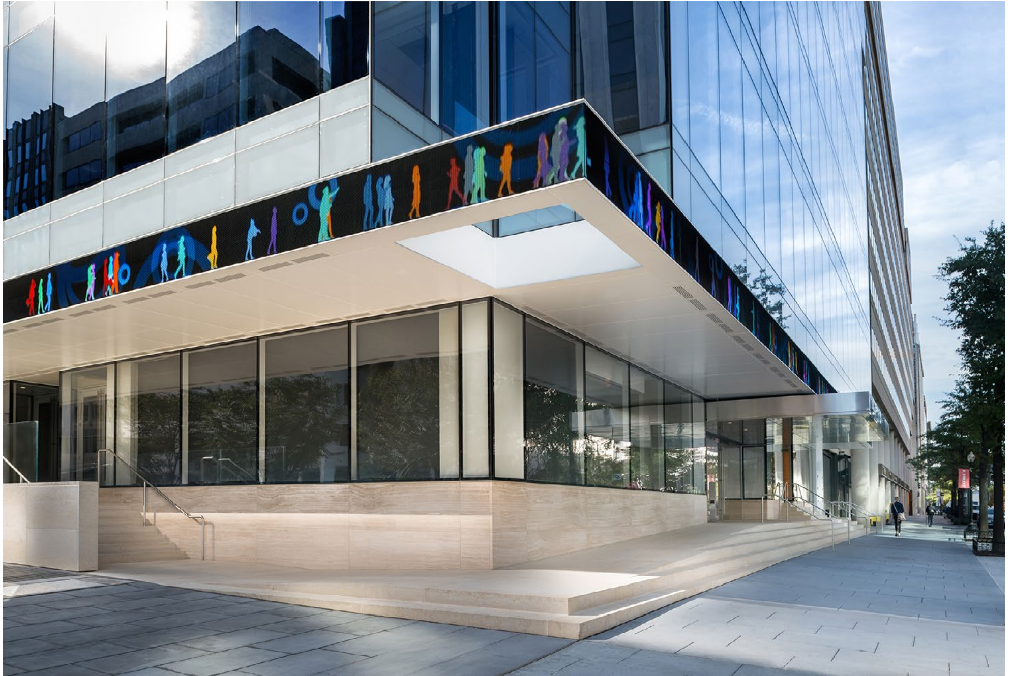
Street level view showing improved pedestrian access
