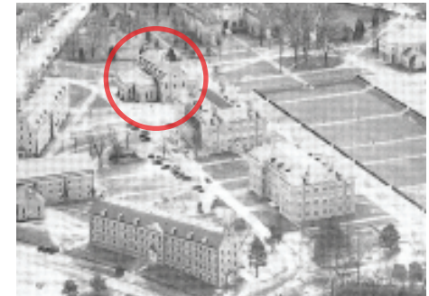
TUCKER HALL WITH 2ND 1929 ADDITION PHOTO /C. 1934
