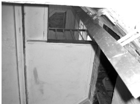
ORIGINAL OBSTRUCTED CUPOLA ABOVE CEILING OF THIRD FLOOR - BEFORE
