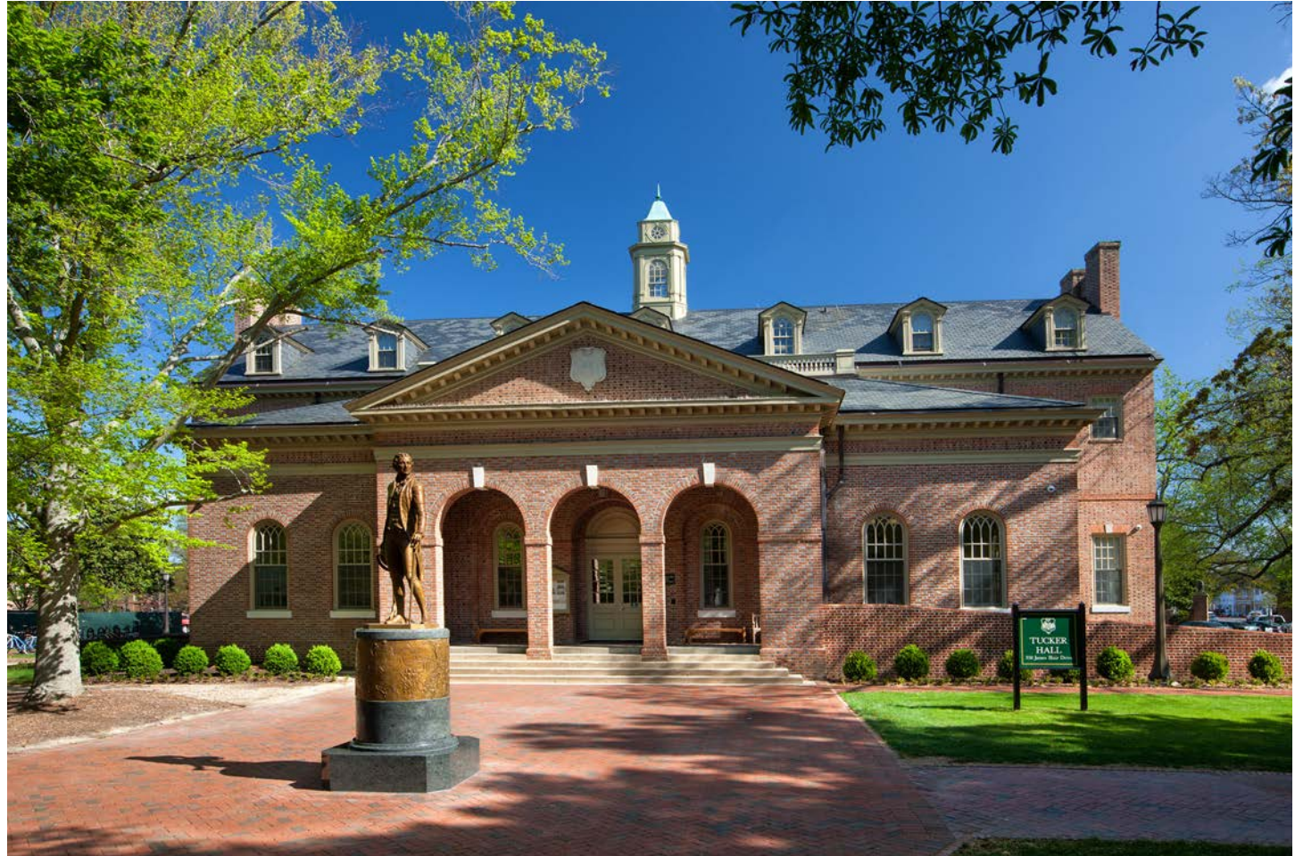
RESTORED TUCKER HALL - AFTER
