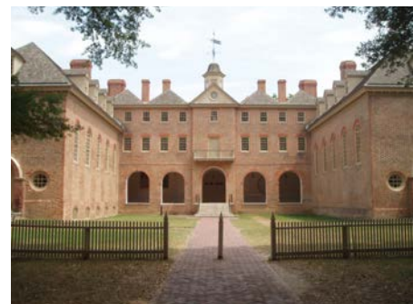
THE HISTORICALLY PROMINENT WREN BUILDING
