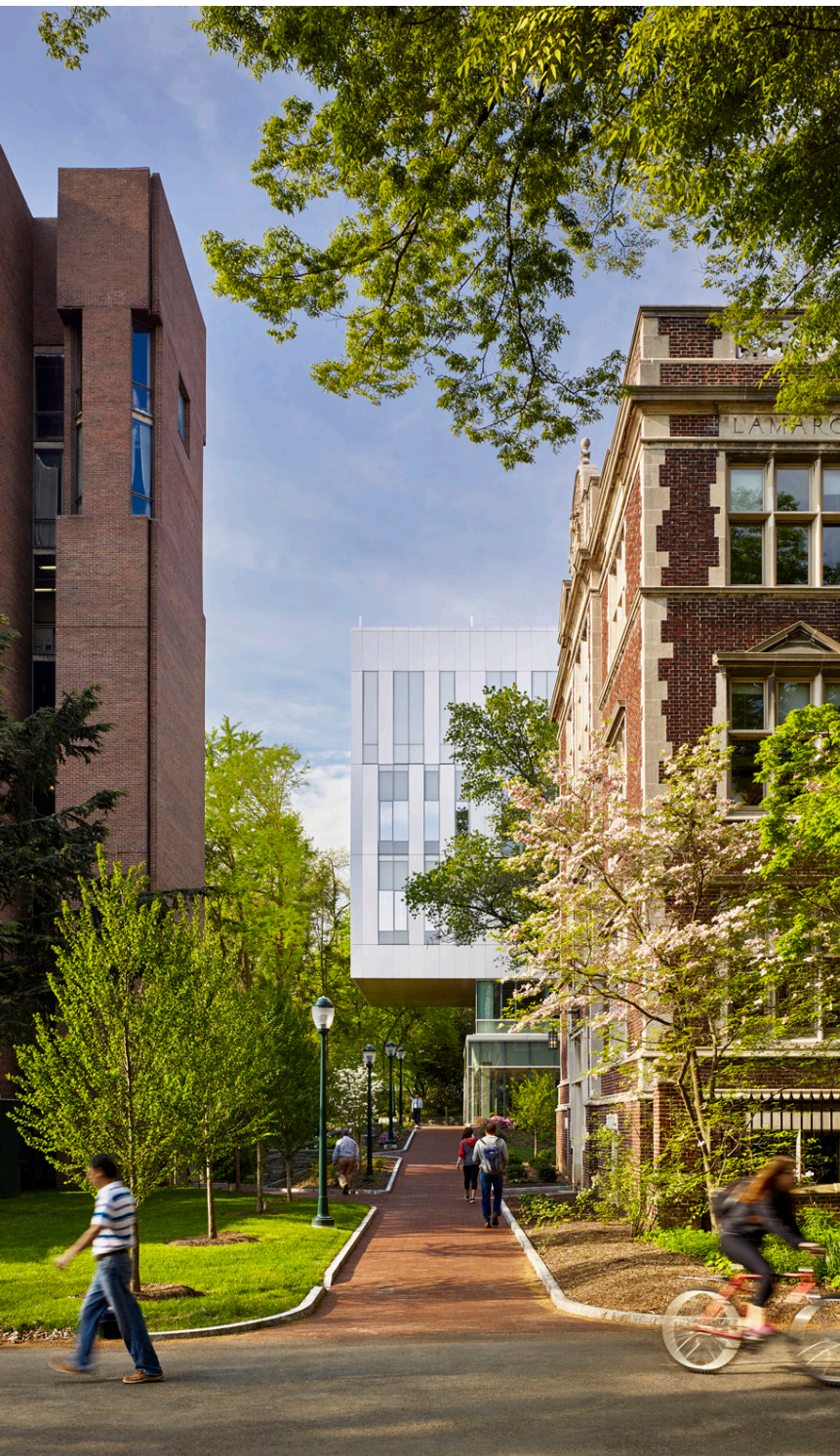
View from Hamilton Walk. The building's east cantilever allowed foundation elements to be pushed back in order to protect the nearby tree roots.
