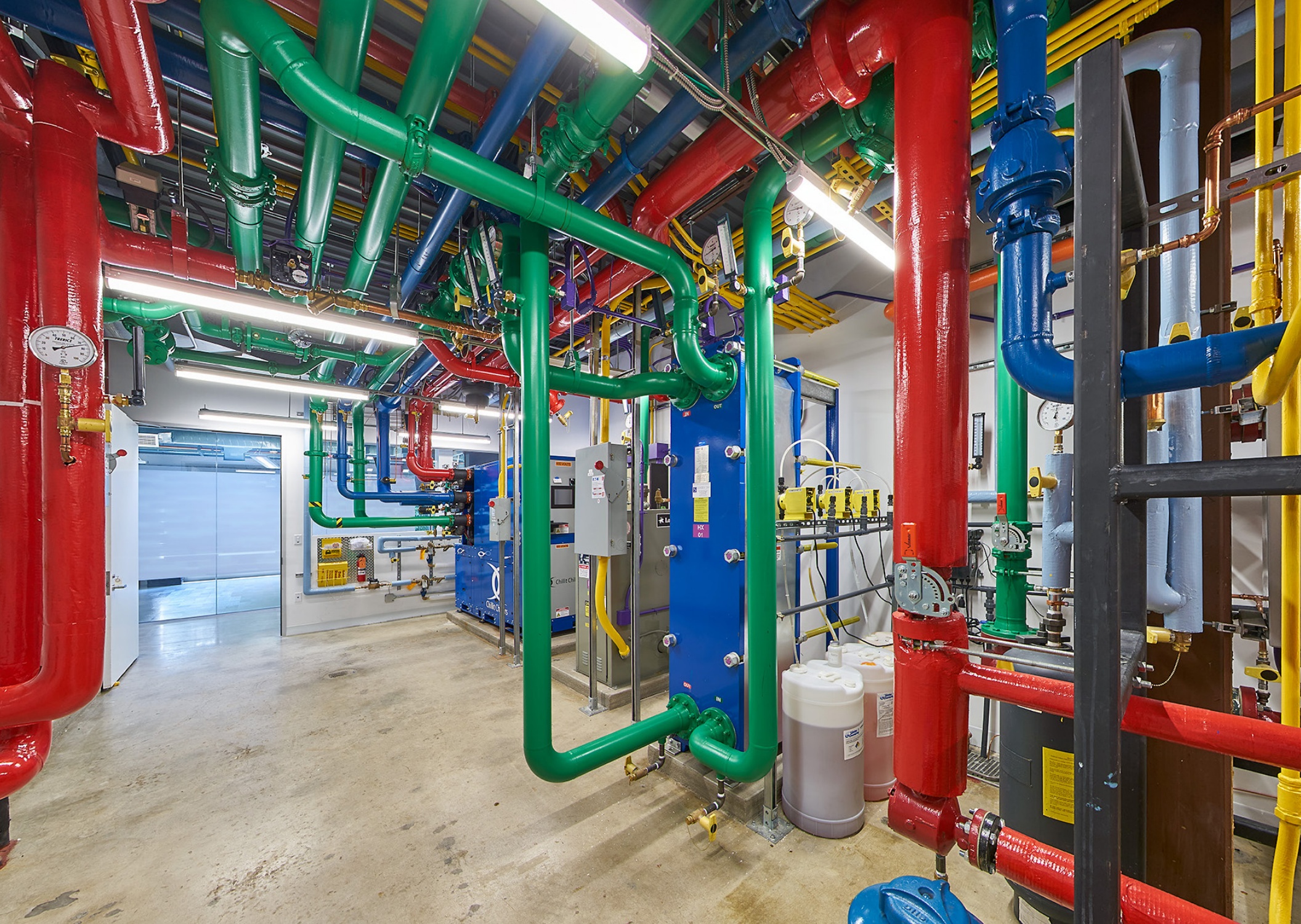
The main mechanical room at DPR Construction's new Headquarters project, targeting net-zero energy, displaying color coded piping for the 6-pipe, heat recovery chiller, the building hot water system with electric boiler and the solar hot water systems for domestic use.
