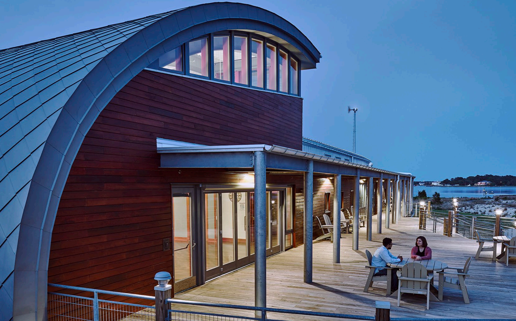
The exterior palette of zinc shingles, sinker-cypress, and galvanized steel reflect the color and forms of the site.
