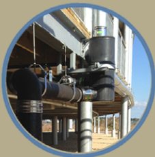
Vortex Filter/First Flush Diverter
