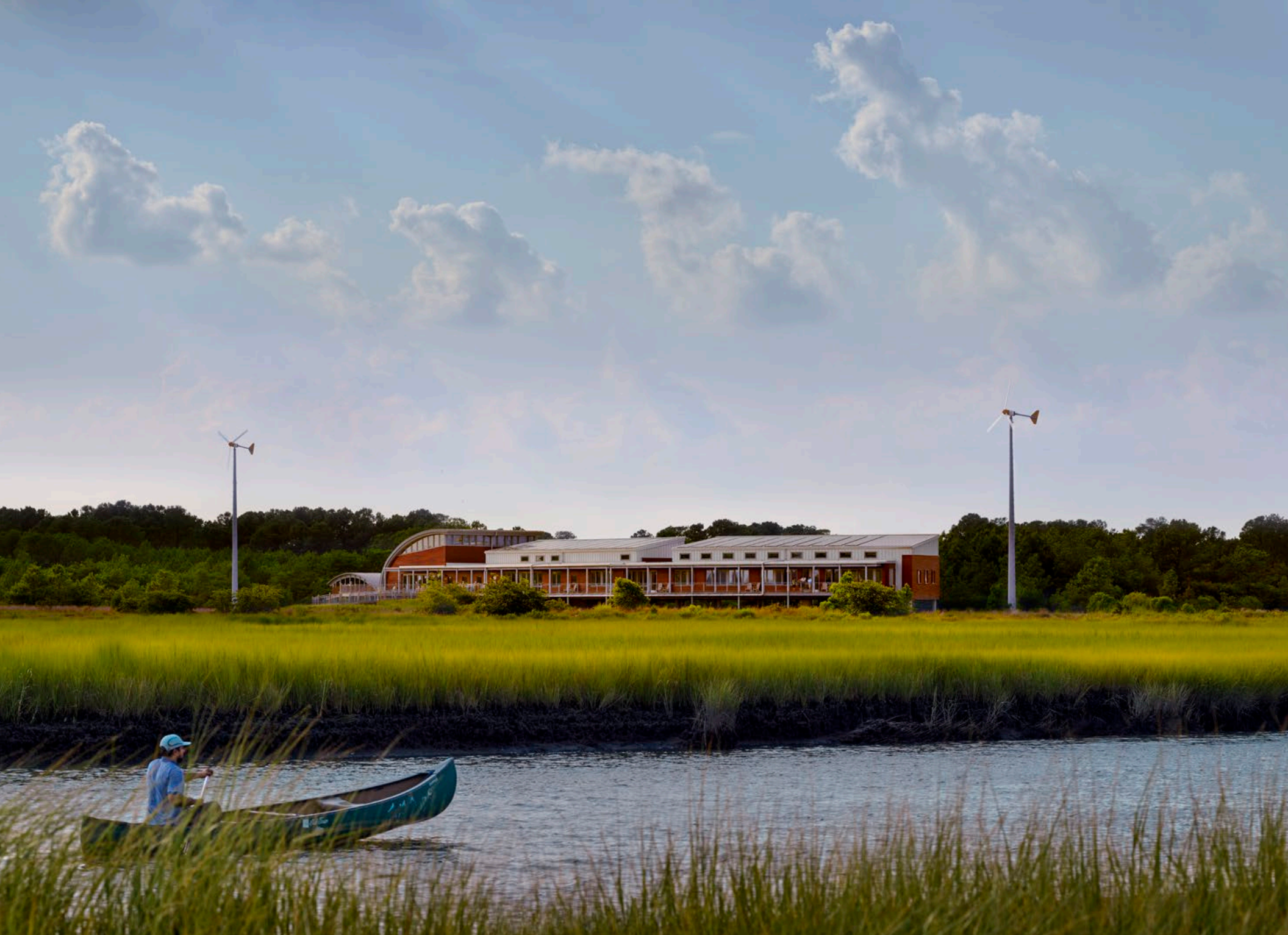
View from the dock looking to the northwest.
