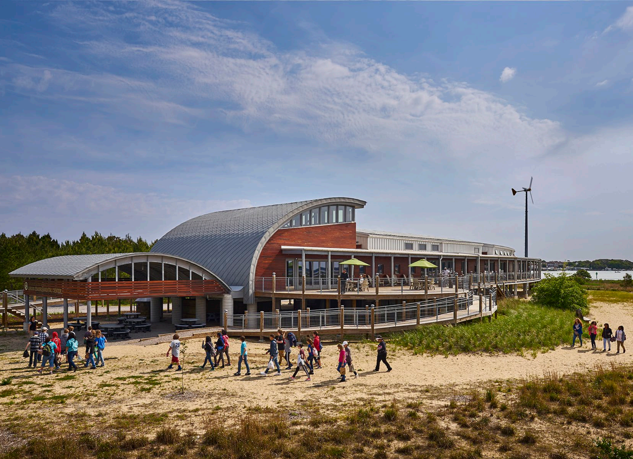
View of the center from the southwest. The Center's low profile and curving forms integrate with its sensitive site.
