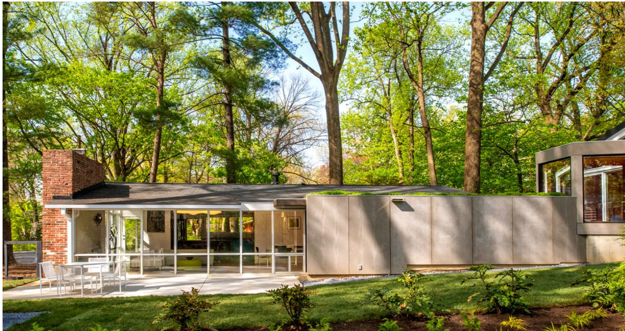
South Elevation of Existing House
