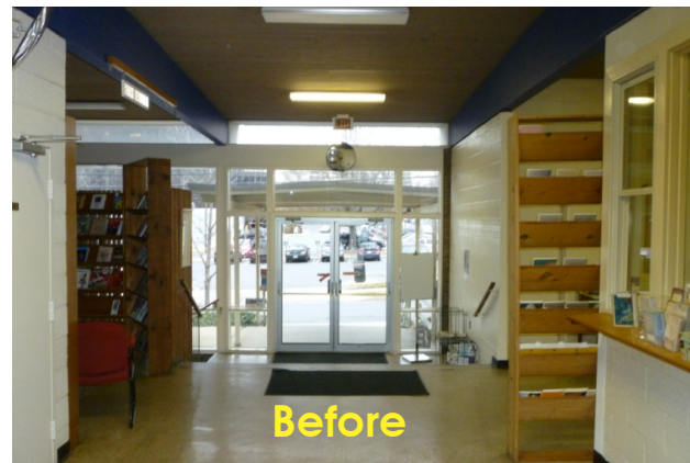
Left - The stair is reconfigured to allow the inclusion of an ADA compliant lift, creating a fully accessible structure
