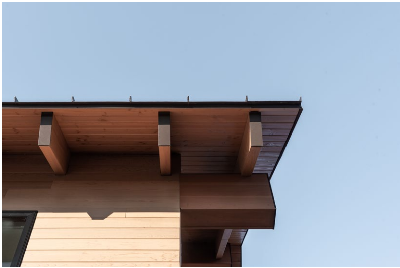
Bathroom, eave, and kitchen details
