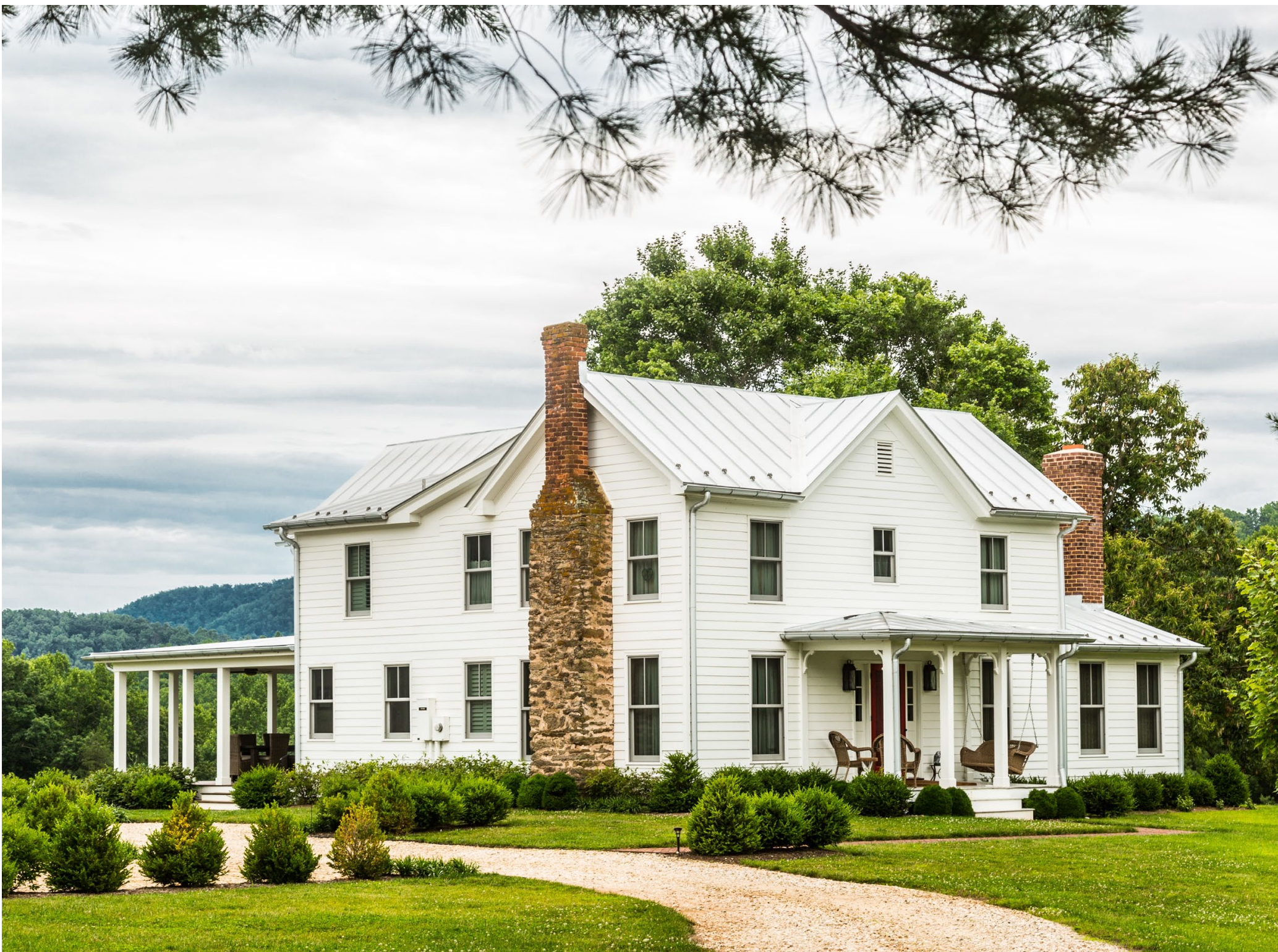
NORTH FACADE OF FARM HOUSE
