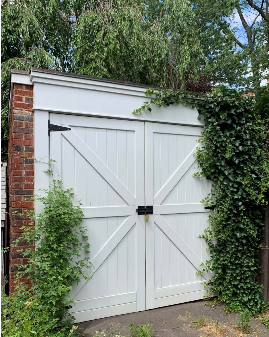
Custom carriage style doors at the driveway side offer access to storage space for outdoor maintenance equipment.
