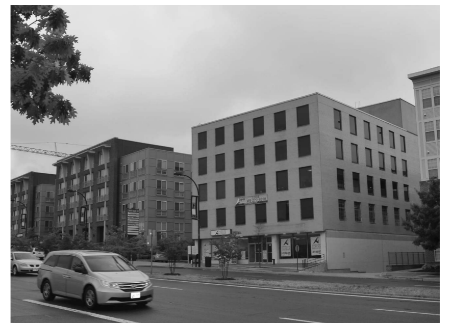
BOTTOM The existing 5-story, 1960s office building LEFT Newly transformed tower, facing northeast across Georgia Avenue
