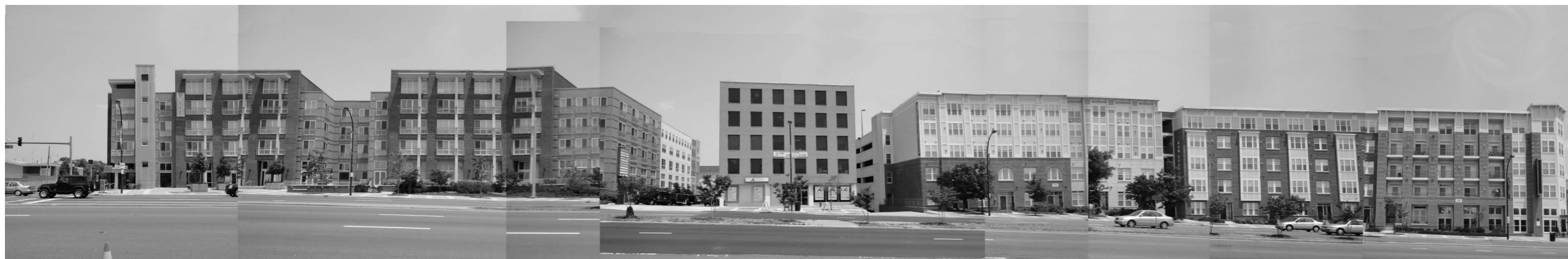
Georgia Avenue skyline facing east BEFORE
