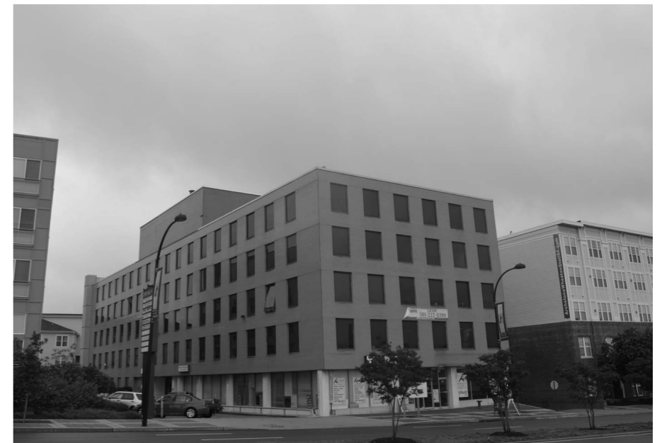
TOP The existing 5-story, 1960s office building
